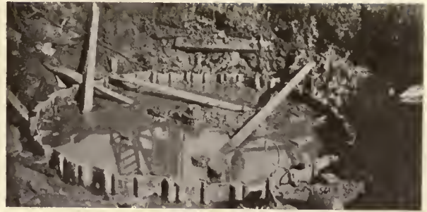
CLOSE-UP OF CYLINDER AFTER DRIVING
