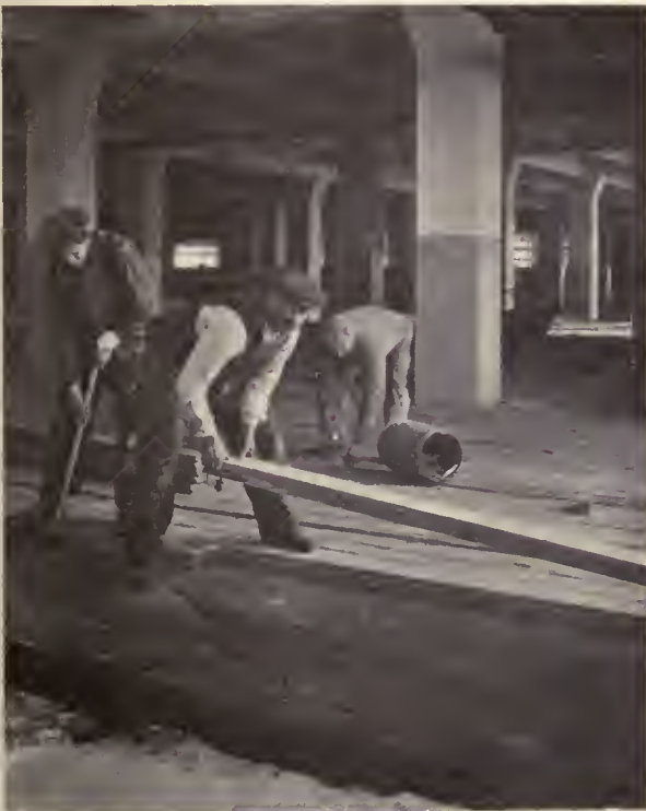
METHOD OF LAYING THE WOOD FLOORING
