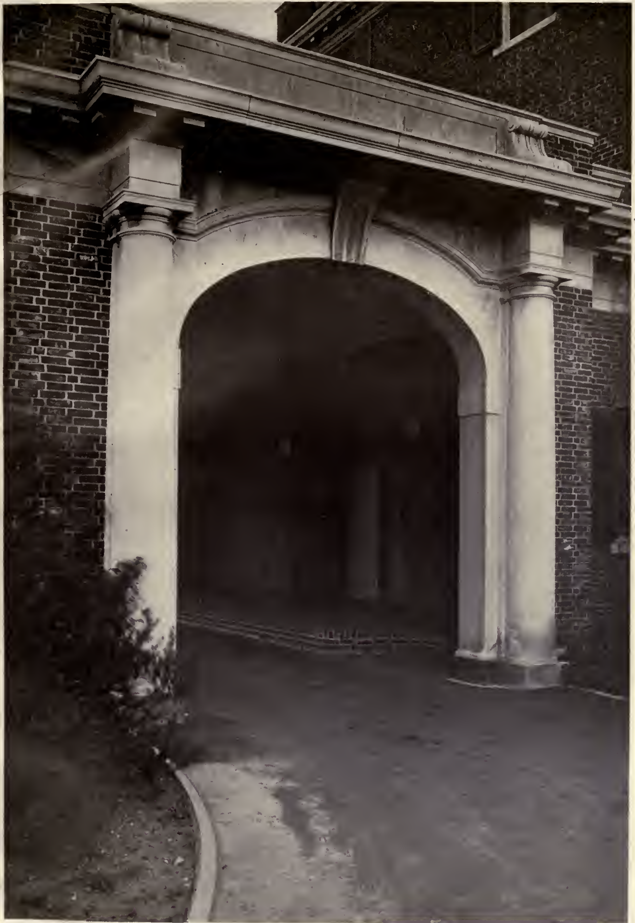
PORTE COCHERE HOUSE OF JAMES J. HILL, OLD WESTBURY, L. I., N. Y. WALKER & GILLETTE, ARCHITECTS
