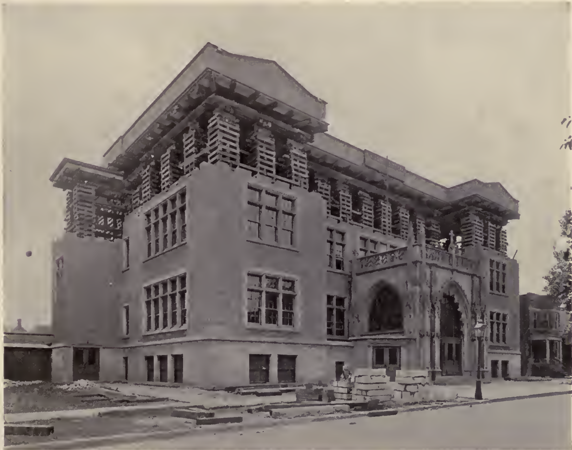
VIEW SHOWING ROOF RAISED AND SUPPORTED
