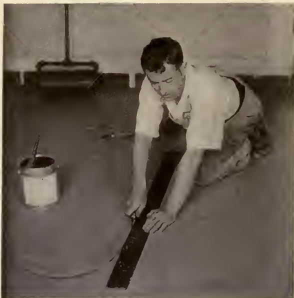
CUTTING JOINTS AND MATCHING SEAMS
