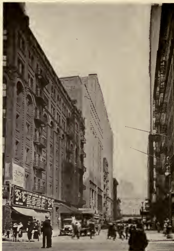
FIG. 9. REAR VIEW OF WURLITZER AND BUSH BUILDINGS, FORTY-SECOND STREET, NEW YORK
