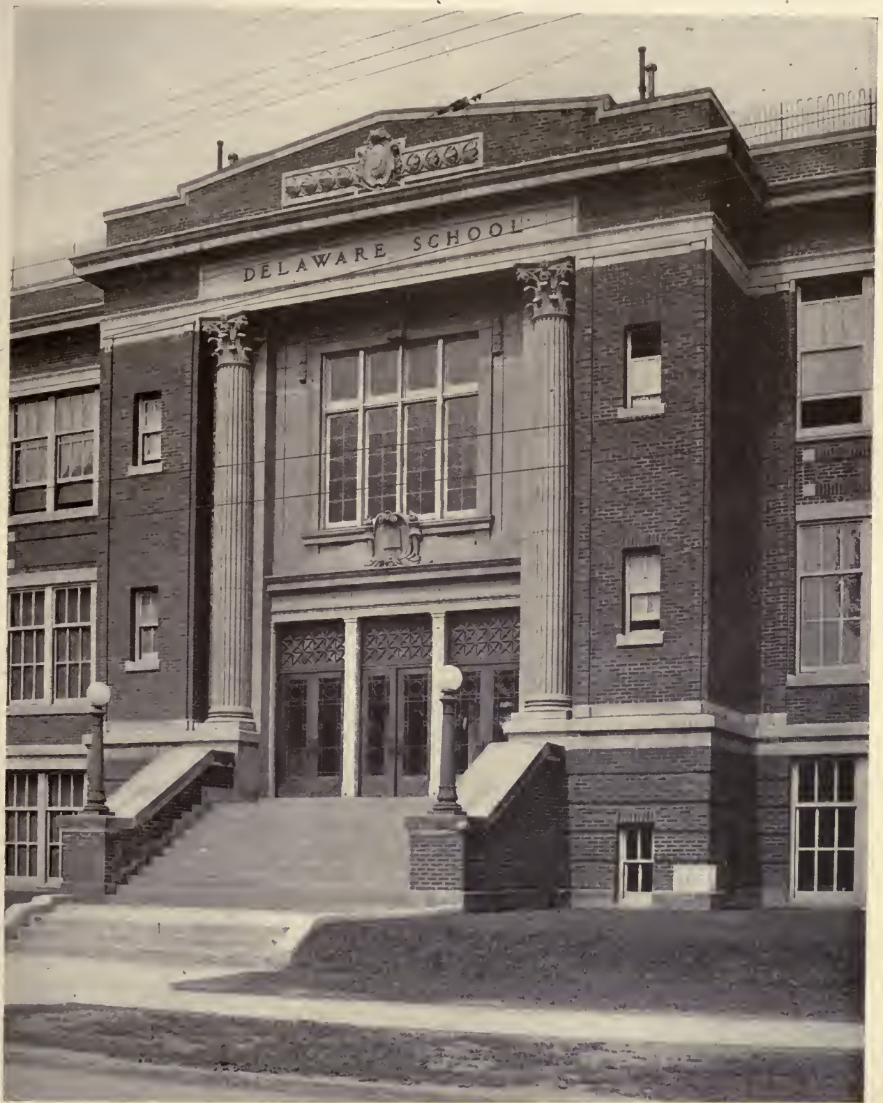
DETAIL OF MAIN ENTRANCE DELAWARE SCHOOL, SYRACUSE, NEW YORK JAMES A. RANDALL, ARCHITECT
