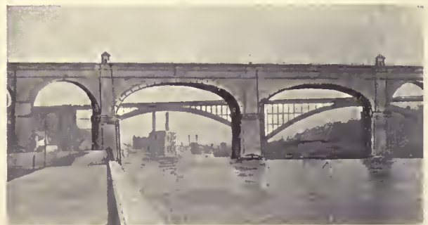
A MODIFICATION OF THE DESIGN OF THE DEPARTMENT OF PLANT AND STRUCTURES WHEREBY THE HORIZONTAL LINES OF THE STEEL GIRDERS ARE "CAMOUFLAGED" TO GIVE THE IMPRESSION OF A MASONRY ARCH.
