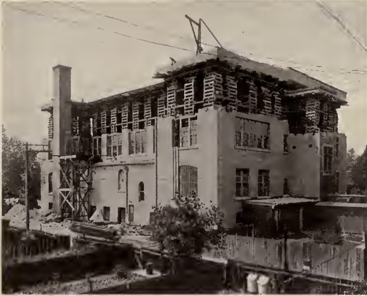
RAISING AND SHORING A FIREPROOF SCHOOL HOUSE
