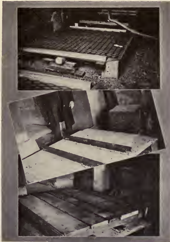
Reinforcement and Supporting Panel in place between concrete supports
