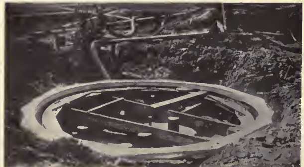
SHOWING TEMPLAT AND CENTER STEEL PIN
