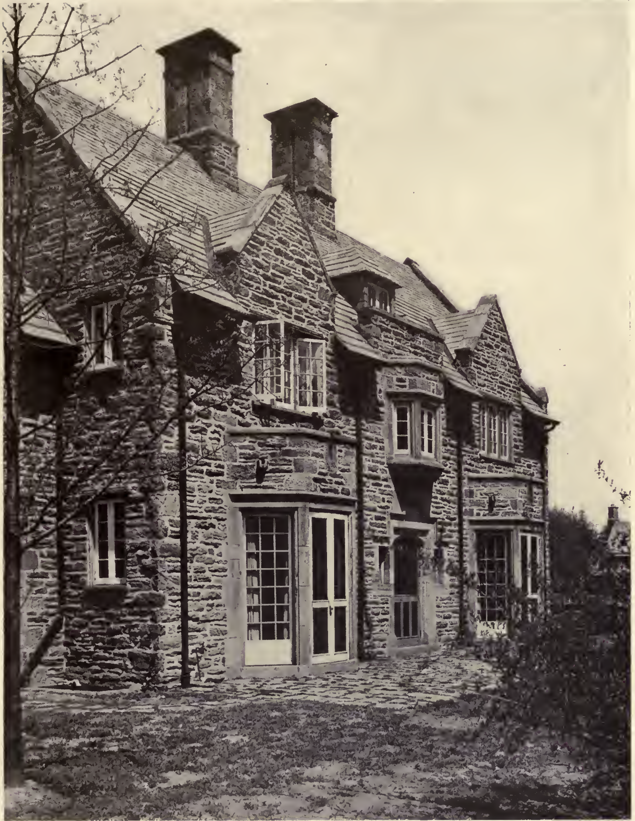
HOUSE OF MR. SPENCER ERWIN, CHESTNUT HILL, PA. ROBERT R. McGOODWIN, ARCHITECT
