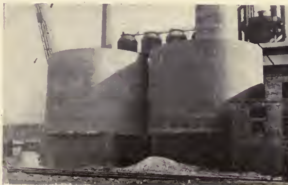
WATER PURIFYING TANKS
