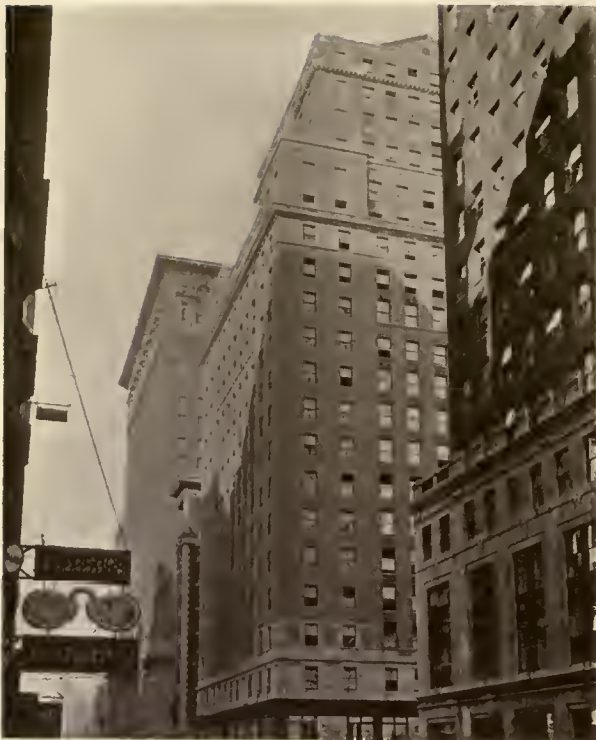
FIG. 3. LIGGETT BUILDING, FORTY-SECOND STREET, NEW YORK
