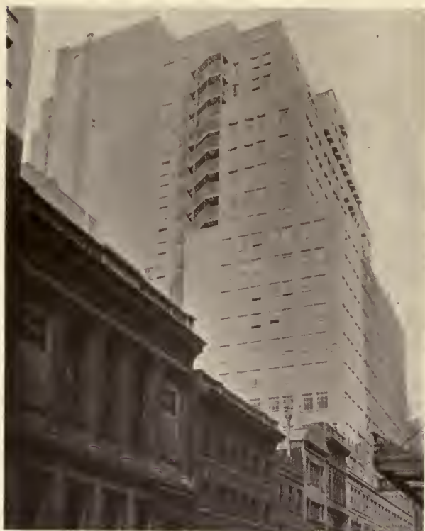
FIG. 8. NATIONAL ASSOCIATION BUILDING, WEST FORTY-THIRD STREET, NEW YORK
