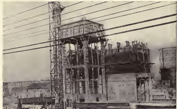
COKE QUENCHING PLANT DURING CONSTRUCTION
