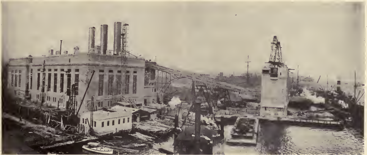
POWER HOUSE—PHILADELPHIA ELECTRIC COMPANY, PHILADELPHIA, PA. The coal unloading tower is seen to the right
