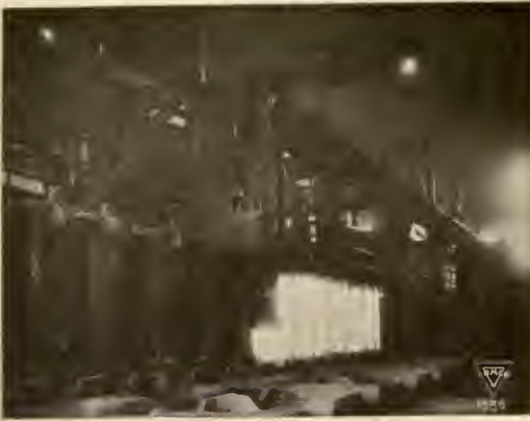
STRIPPING MOLDS FROM THE INGOTS
