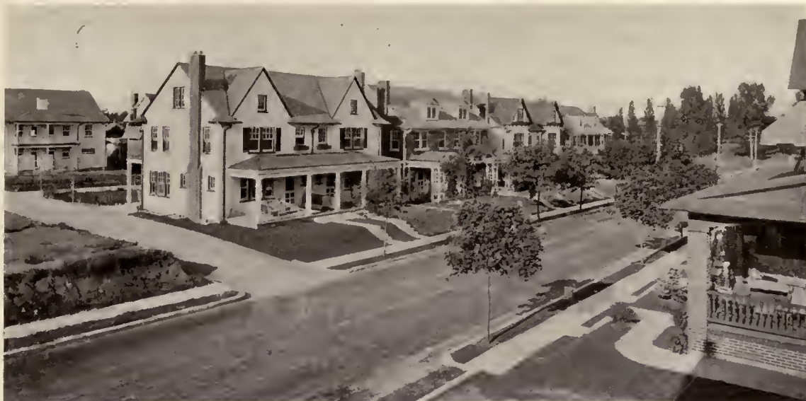
GROUP OF HOUSES AT LANCASTER, PA., IN WHICH LINOLEUM IS USED FOR ALL FINISHED FLOORS THROUGHOUT EACH HOUSE
