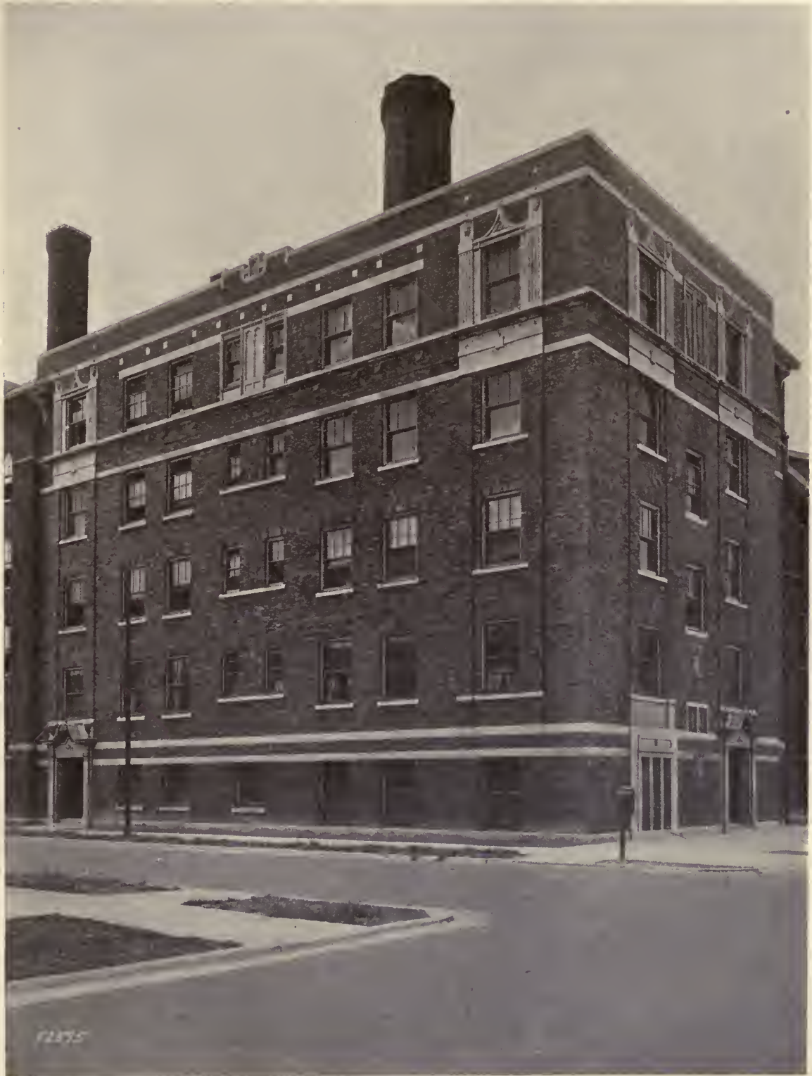
DORMITORY "C" AND BOILER HOUSE BETHANY BIBLE SCHOOL, CHICAGO N. MAX DUNNING, ARCHITECT
