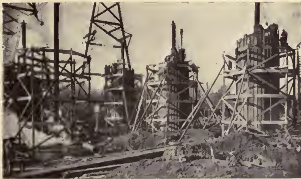
CYLINDERS ASSEMBLED FOR DRIVING
