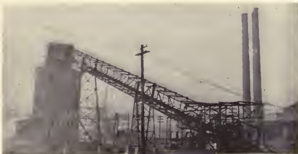
COAL MIXING AND PULVERIZING PLANT, SHOWING STEEL LOADING TRESTLE
