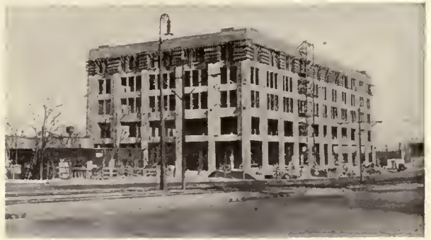
STRUCTURAL FRAME COMPLETED
