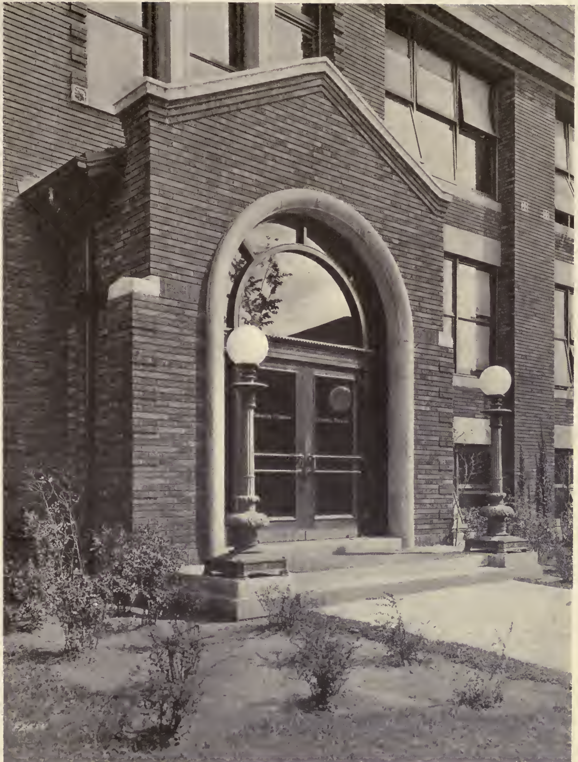
ENTRANCE DETAIL OFFICE BUILDING FOR SIMMONS MANUFACTURING COMPANY, KENOSHA, WIS. N. MAX DUNNING, ARCHITECT
