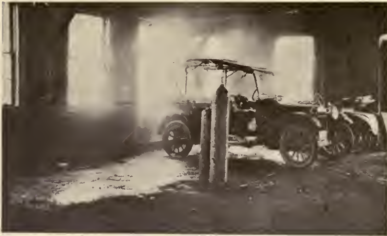
FIG. 1. FIRE EXTINGUISHED BY ONE SPRINKLER HEAD, WHICH WAS STILL OPERATING WHEN THIS PICTURE WAS TAKEN
