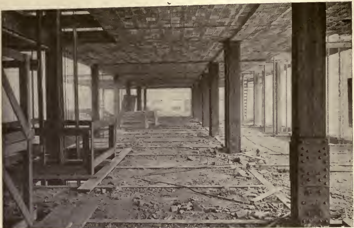
INTERIOR VIEW DURING CONSTRUCTION, OLD COLONY LIFE BUILDING, CHICAGO, ILL.
