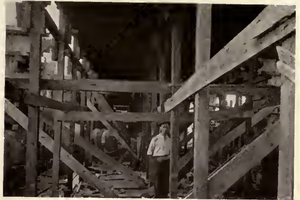
FIG. 3. VIEW UNDER SUPPORTS
