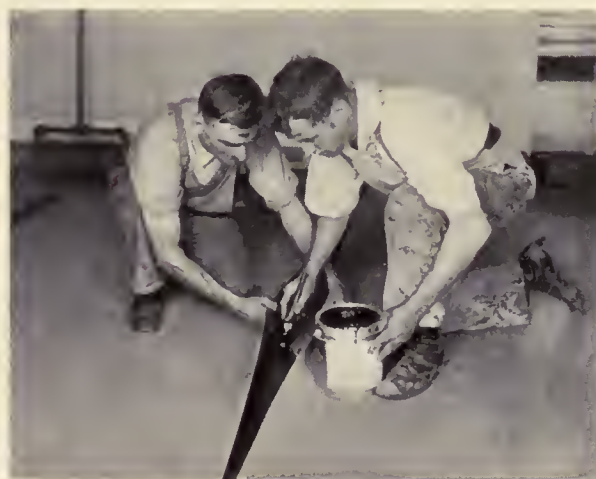
APPLYING CEMENT TO THE FELT
