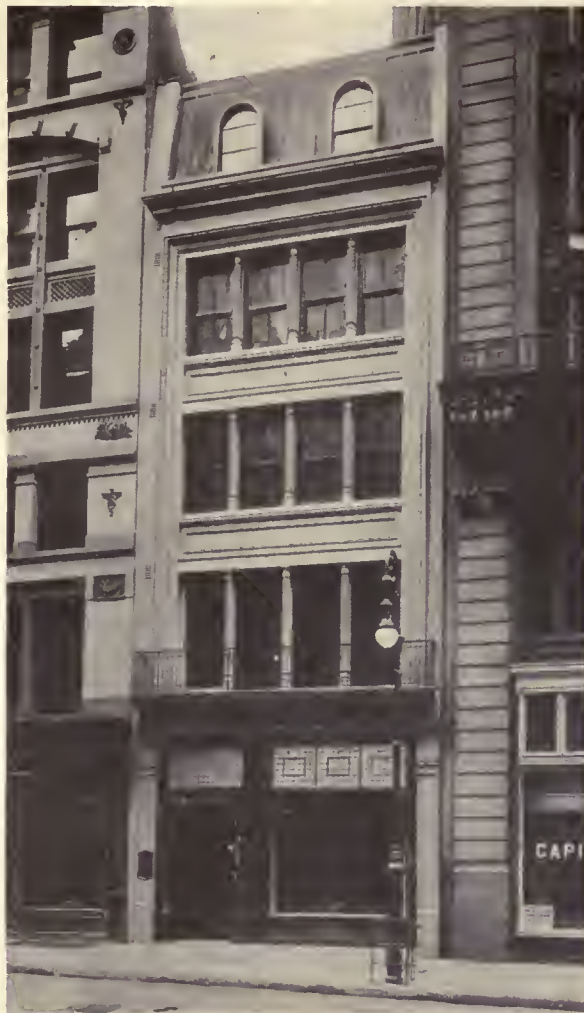
EXTERIOR OF BUILDING AFTER REMODELING
