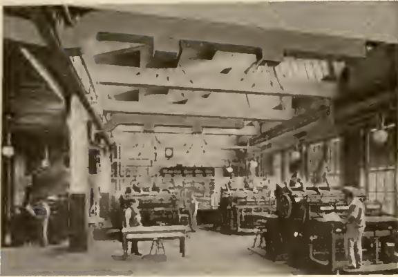
HOT-BLAST SYSTEM INSTALLED IN PRINTING ESTABLISHMENT
