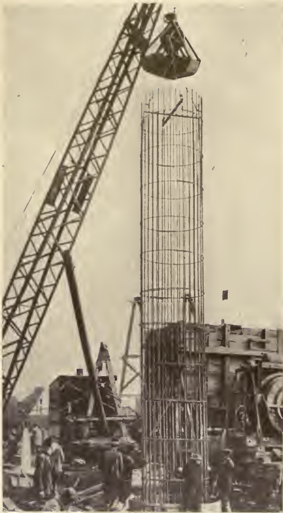
PLACING REINFORCED STEEL CAGE IN CYLINDRICAL WELL
