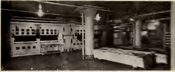
VIEW IN BAKERY DEPARTMENT ON SECOND FLOOR
