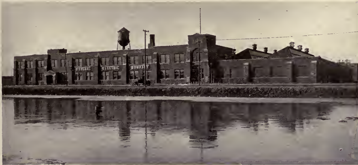
BUILDING FOR FEDERAL ELECTRIC CO., CHICAGO, ILL. GEORGE C. NIMMONS & CO., ARCHITECTS
