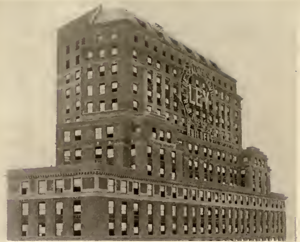
FIG. 5. UPPER STORIES OF FISK BUILDING
