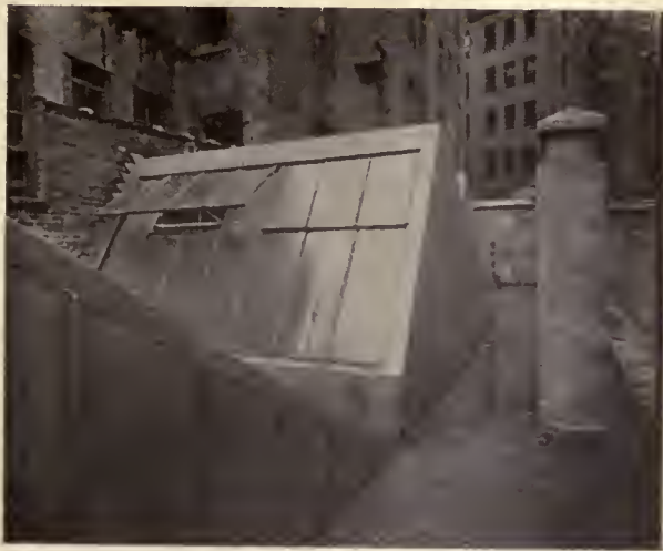
SAW-TOOTH ROOF WHICH REPLACED OLD SKYLIGHTS
