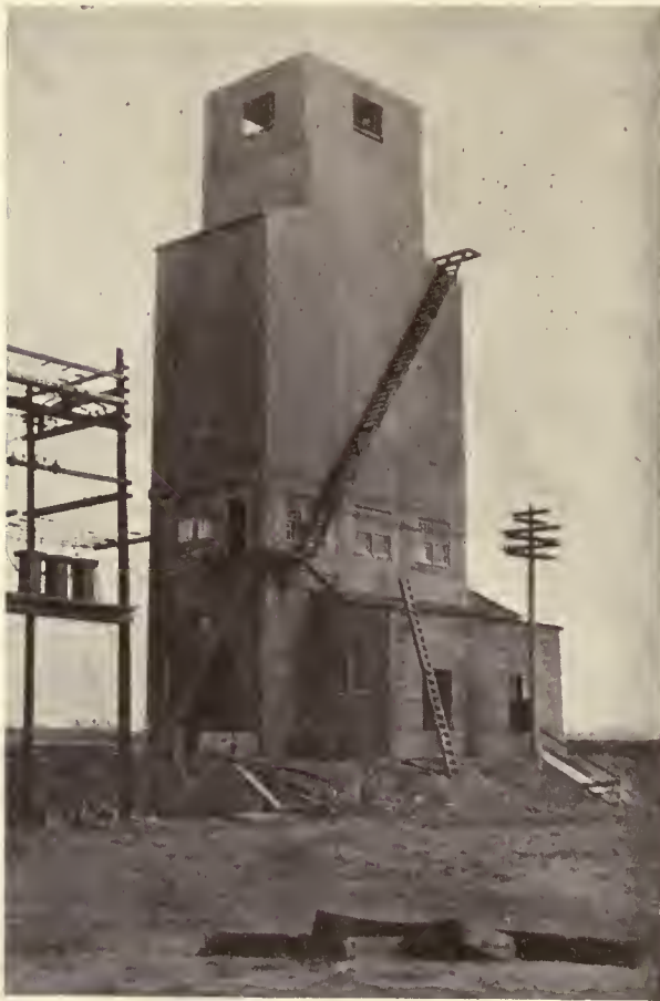
COAL MIXING AND PULVERIZING PLANT DURING CONSTRUCTION
