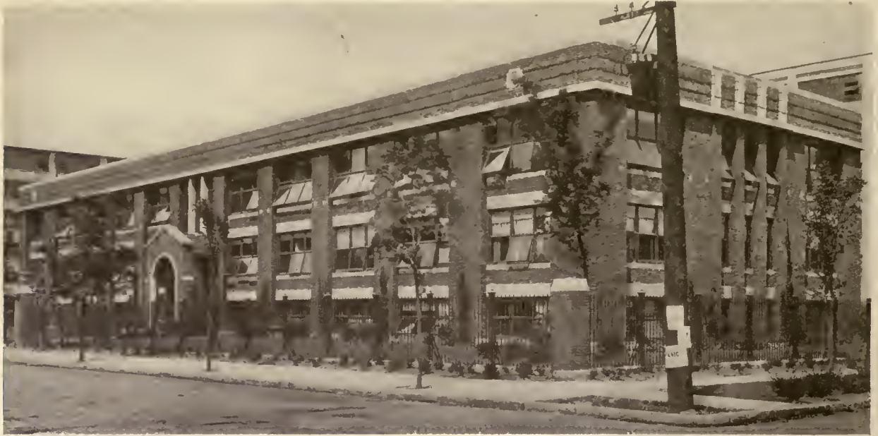
OFFICE BUILDING FOR SIMMONS MANUFACTURING COMPANY, KENOSHA, WIS. N. MAX DUNNING, ARCHITECT
