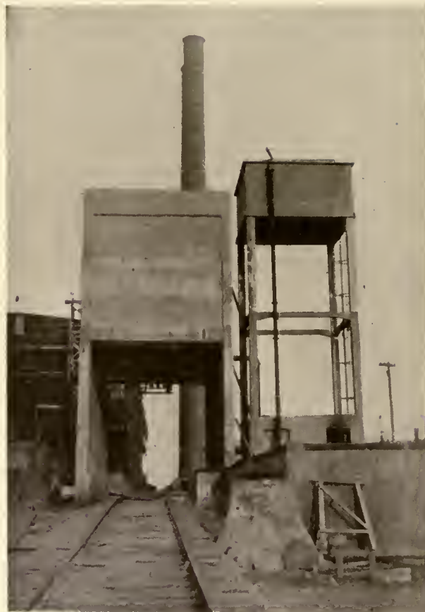
COKE QUENCHING PLANT
