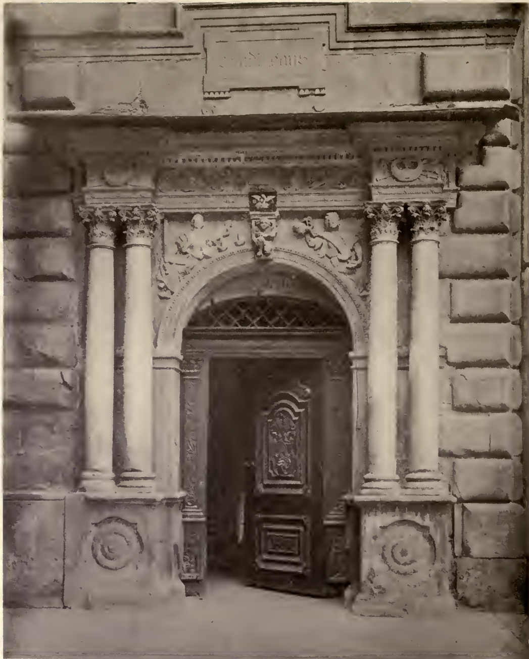
DETAIL OF DOORWAY—RATHAUS, LUCERNE
