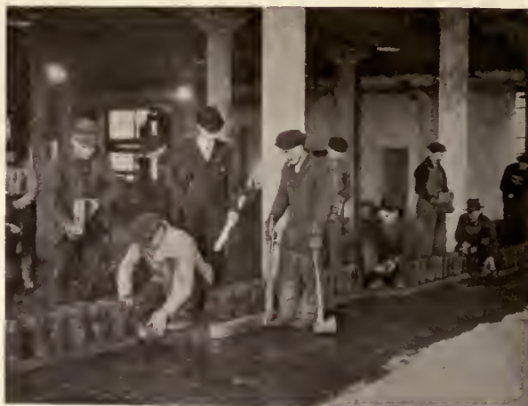
LAYING A WOOD BLOCK FLOOR
