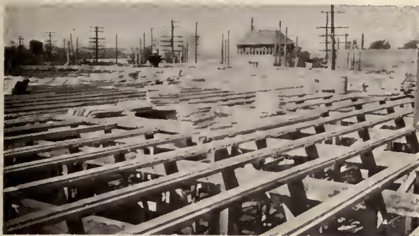
FLOOR FORMS UNDER CONSTRUCTION
