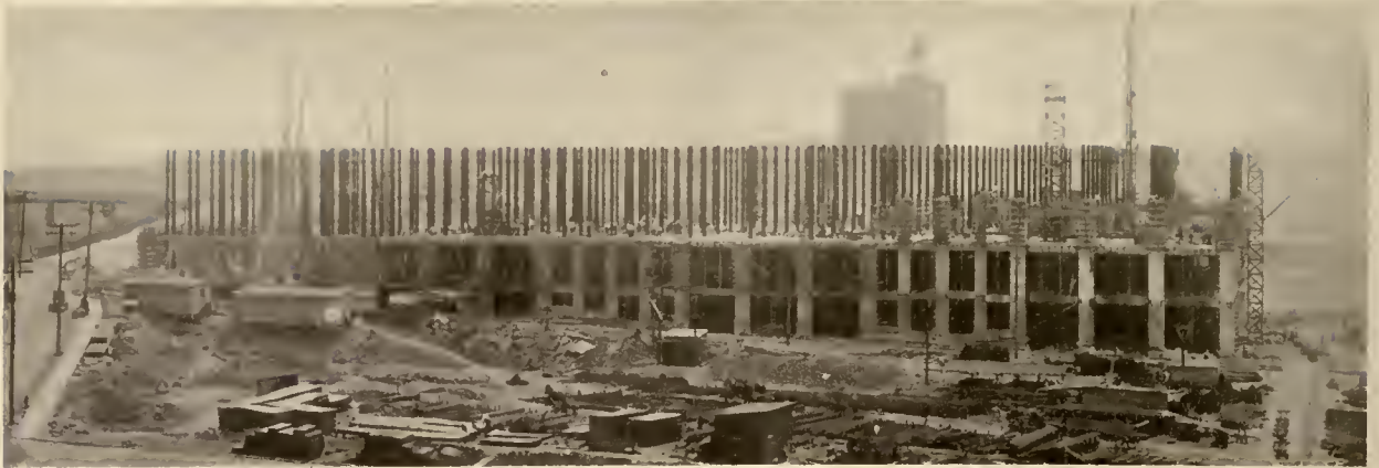
PROGRESS VIEW Showing erection of steel columns
