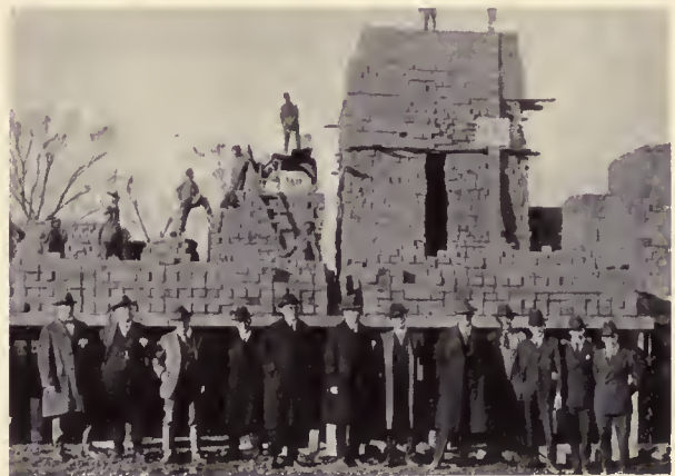
CLOSE-UP OF PANEL H UNDER LOAD
