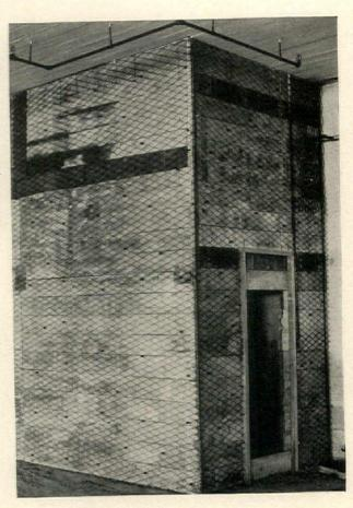
Forms previously used for flat slab floor construction, in place for partitions about the toilet rooms
