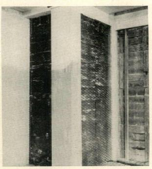
Forms covered with tar paper and reinforcement, in place in wall enclosing chimney
