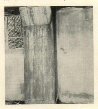
Hollow Gunite wall with finish coat and unfinished concrete column
