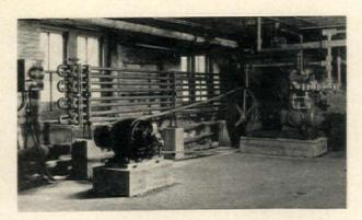
Refrigerating Plant, with Compressor, Condenser, Receiver and Electric Cabinet
