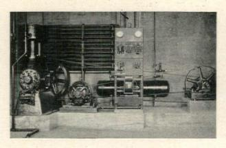
Refrigerating Plant, Showing Compresor, Condenser, Receiver and Switch and Gauge Board
