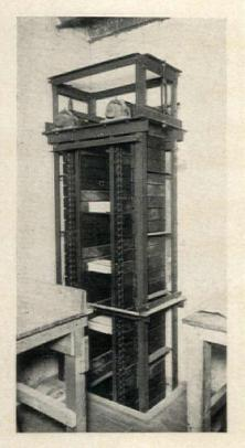
Top of a Subveyor Before the Enclosing Partition is Installed
