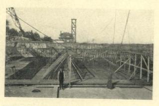
REINFORCING PARTIALLY IN PLACE IN THE 9'-0" THICK PORTION OF THE FOUNDATION
