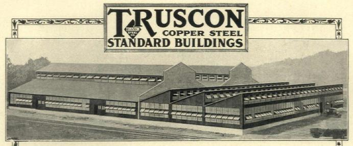
IRONTON STOVE & MANUFACTURING CO., IRONTON, OHIO A factory group combining Sawtooth and Type 3-M Truscon Standard Buildings.
