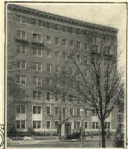
PFTS, 1724 17TH ST. N.W. WASHINGTON, D. C. Architects Stern & Tomlinson Builder, Howard Eckison
