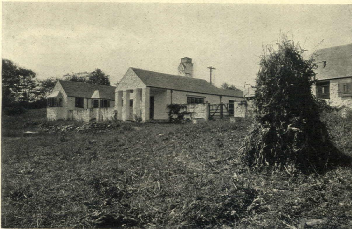
AN INTERESTING EXAMPLE OF A MODERN FARM GROUP DESIGNED BY ALFRED HOPKINS, ARCHITECT
