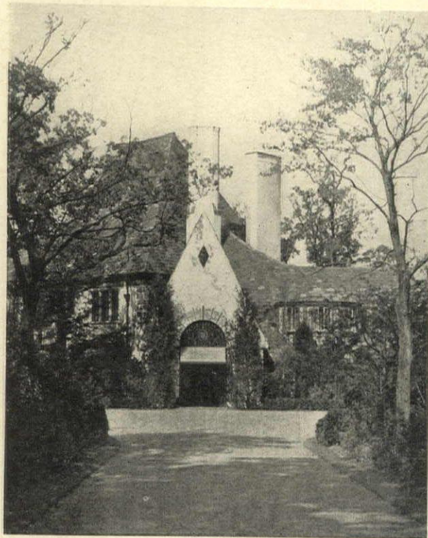
APPROACH FRONT HOUSE OF MRS. CLYDE CARR, FOREST LAKE, ILL. H. T. LINDBERG, ARCHITECT
