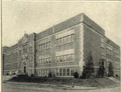
DE LASALLE SCHOOL, MINNEAPOLIS, MINN. Architects, Damon, O'Meara & Hills Contractor J. A. McDonald Construction Co.
