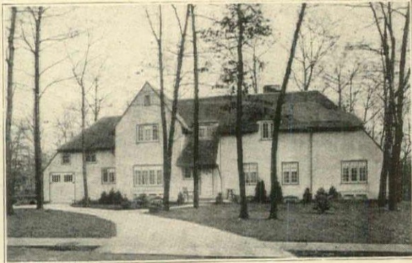
Residence of Geo. W. Klewer, Architect, 36 Crescent Drive, Glencoe, Ill. Bishopric Sheathing used as sub-flooring, on roofs under shingles, and as Sheathing under Bishopric Stucco-Base. Bishopric Base used on all exteriors. Bishopric Plaster Base used on all interiors
