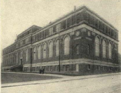
OMAHA TECH. HIGH SCHOOL, OMAHA, NEB. Architects, Frederick W. & Edwin B. Clarke Contractors, F. P. Gould & Sons
