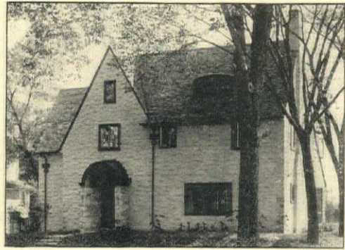
Chicago common brick finished with Cabot's Old Virginia White; roof stained with Cabot's Shingle Stain. Lowe & Bollenbacher, Architects, Chicago
