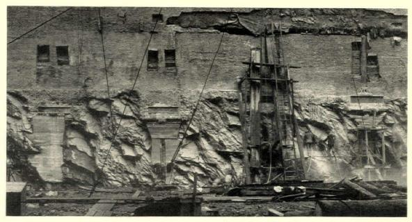
VIEW OF WEST WALL OF PRESENT BUILDING, SHOWING STEEL STRUT AND CONCRETE UNDERPINNING OF EXISTING FOUNDATIONS. HEAVY TIMBER SHORES USED TO PREVENT LATERAL MOVEMENT OF THE EXISTING COLUMNS
