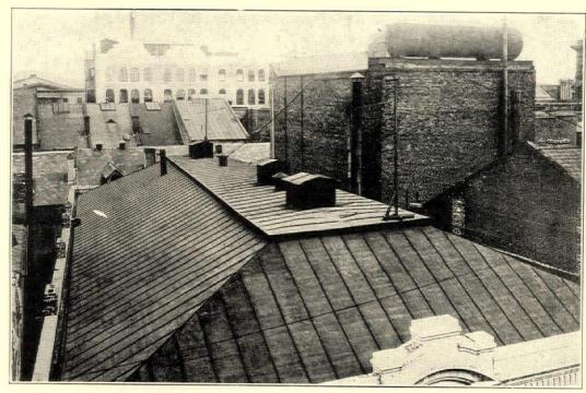
This is an ARMCO-Ingot Iron Roof on the Old Sazerac Building, New Orleans. It has already seen fifteen years of service.
