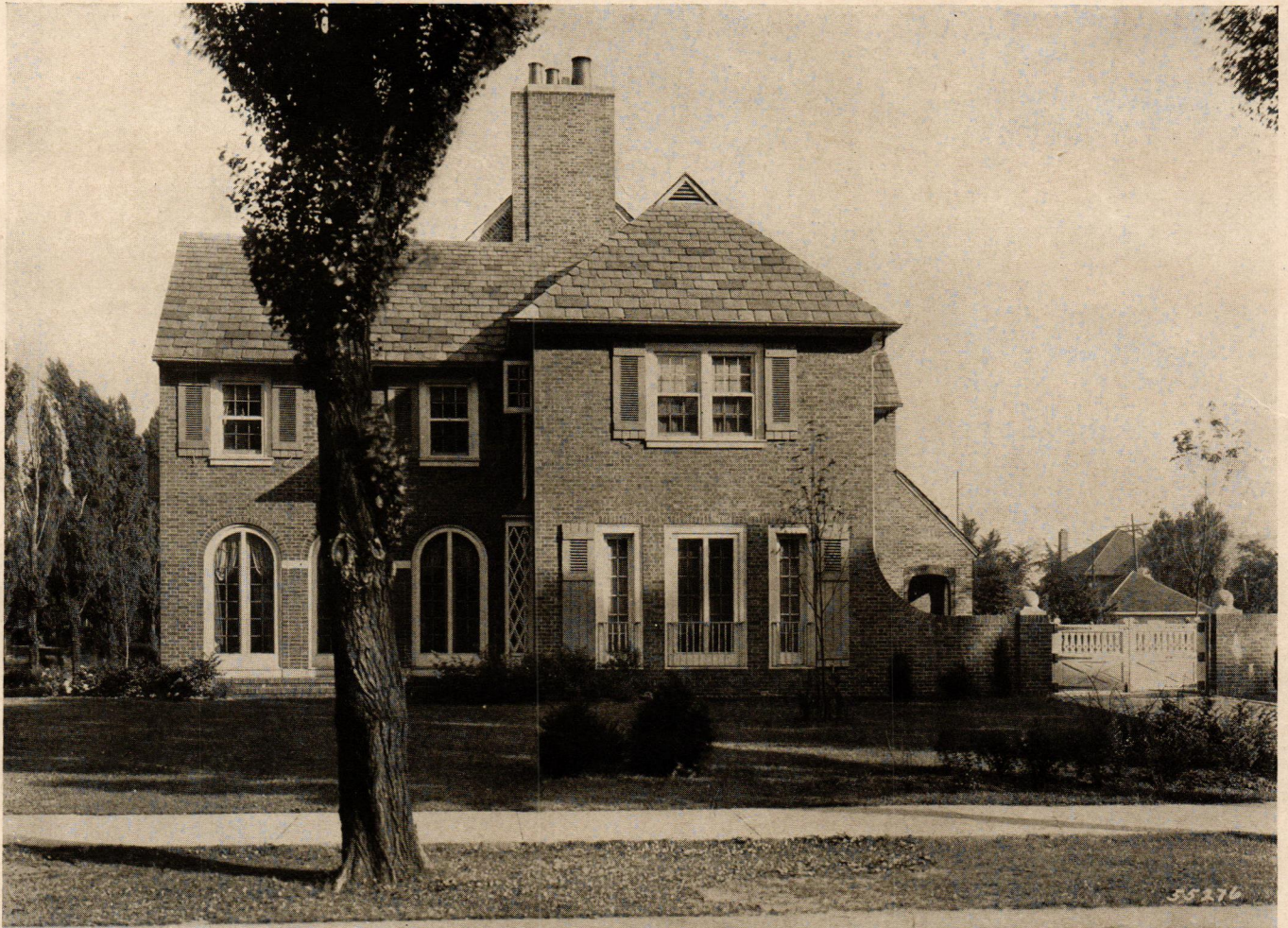
HOUSE OF LYFORD MOORE, DETROIT, MICH. J. IVAN DISE, ARCHITECT—E. J. MAIER, ASSOCIATE
