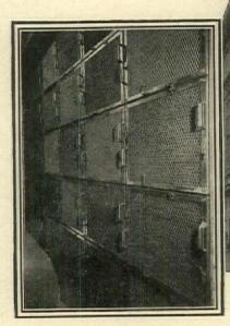
The above illustrations show Lord & Taylor's store, Fifth Avenue, New York City, and the installation of Reed Air Filters that provides 30,000 cubic feet of clean air a minute for restriction. clean air a minute for ventilation.
