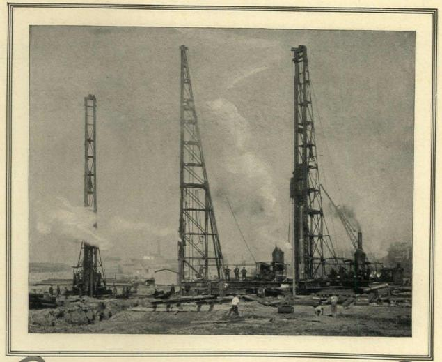
RAYMOND Composite (Wood Concrete) Piles not only join timber to concrete in such a way that the transverse strength at any section approximates that of the wood pile . . . . they accomplish this result by a method that permits inspection and checking of each step.
