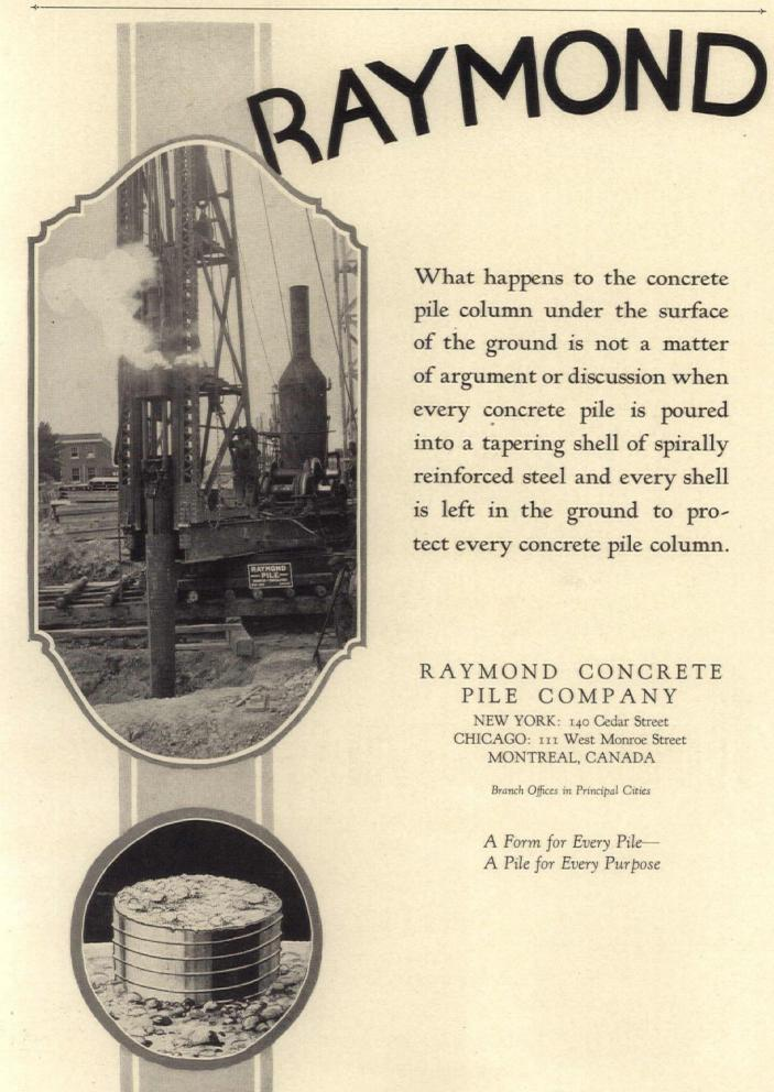
What happens to the concrete pile column under the surface of the ground is not a matter of argument or discussion when every concrete pile is poured into a tapering shell of spirally reinforced steel and every shell is left in the ground to protect every concrete pile column.
