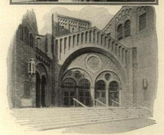
THE high quality of the center pivoted type of Truscon Steel Windows is evidenced by their selection for the Moody Church, Chicago. A pleasing effect in thorough harmony with the excellence of the building is obtained with a very economical type of Truscon Steel Window.
