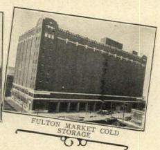
THE ABOVE STRUCTURES are reinforced throughout with RAIL STEEL BARS
