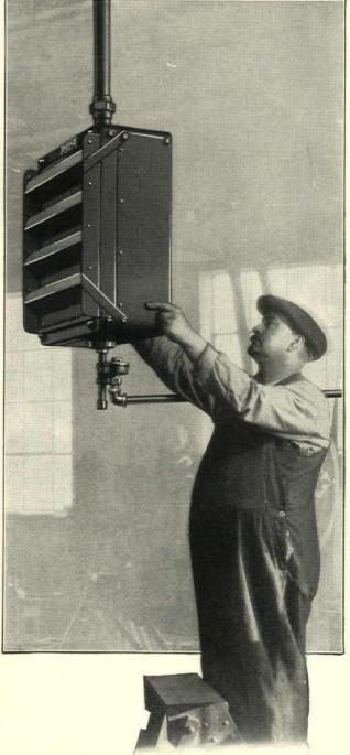
The illustration shows how simple it is to DIRECT THE HEAT from the Modine Unit Heater WHERE NEEDED — toward a bad door or window, lathe, work benches, etc. One man with a wrench does it in a few minutes' time.
