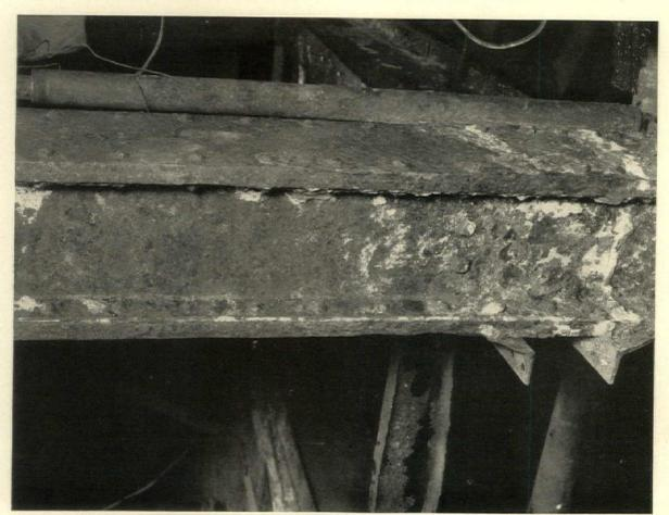
BOILER AND COAL ROOM WHERE WATER RAN OVER SLACK ILLINOIS BITUMINOUS COAL. DISSOLVED ACIDS PENETRATED THE FIREPROOFING AND DESTROYED THE PROTECTIVE PAINT ON THE STEELWORK, CAUSING CORROSION OF THE STEELWORK. UNDER THESE CONDITIONS STEEL MUST BE PROTECTED WITH AN ACID-PROOF COATING, AND THE FIREPROOFING EITHER OF TILE OR CONCRETE MUST BE ABSOLUTELY WATERPROOF AND ACID-RESISTING. NO CORROSION FOUND IN OTHER PARTS OF THE STRUCTURE
