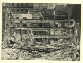
FORREST THEATRE. PHILADELPHIA, ERECTED IN 1905. DEMOLISHED IN 1927. STEELWORK WAS FOUND TO BE FREE FROM CORROSION
