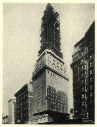
TOWER BUILDINGS MAKE THE MATTER OF WIND BRACING CONNECTIONS OF UNUSUAL IMPORTANCE. COLUMN BEARINGS, ALWAYS IMPORTANT, TAKE ON RENEWED IMPORTANCE IN BUILDINGS OF THIS TYPE. THE ABOVE ILLUSTRATION INDICATES THE STRUCTURAL PROBLEMS INVOLVED IN SETBACK STRUCTURES. INSPECTION PRINCIPLES ARE THE SAME FOR TOWER BUILDINGS AS FOR OTHERS
