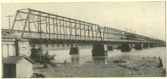
SUSQUEHANNA RIVER BRIDGE AT HAVRE DE GRACE, MD. OPENED FOR RAILROAD TRAFFIC IN 1878 BY THE PENNSYL-VANIA RAILROAD COMPANY. CONVERTED TO A HIGHWAY TOLL BRIDGE IN 1910. AN UPPER DECK ROADWAY INSTALLED FOR TWO-WAY TRAFFIC IN 1927. ORIGINAL METAL IN PERFECT CONDITION
