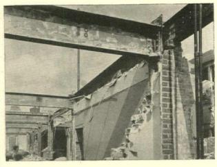
BLENHEIM APARTMENTS, PHILADELPHIA, ERECTED IN 1901, DEMOLISHED IN 1927. STEELWORK AS CLEAN AND IN AS GOOD CONDITION AS WHEN FIRST ERECTED
