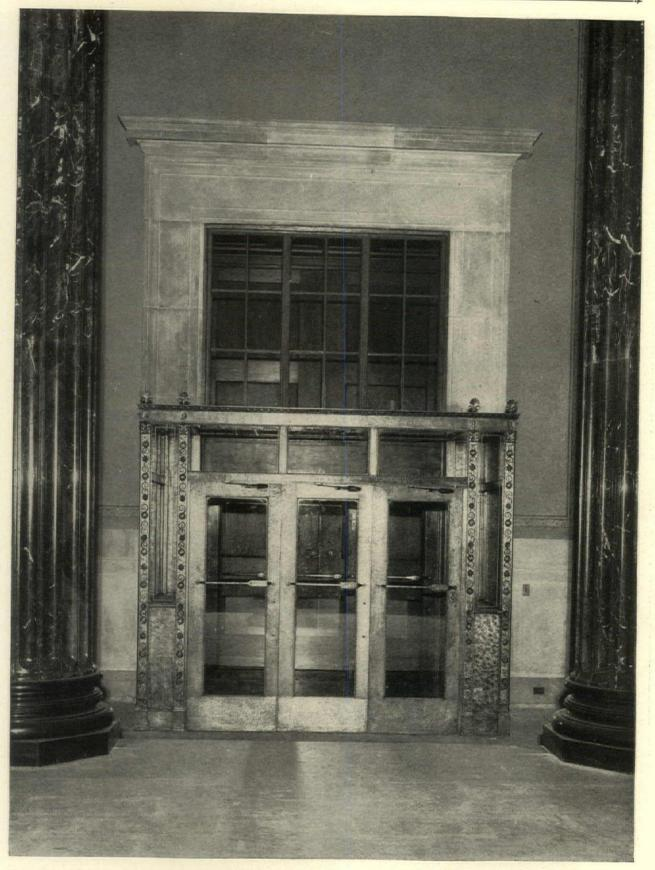
THE ENTRANCE IS OF WROUGHT IRON IN INTERESTING DESIGN. THE CASING OF THE DOOR OPENING IS OF INDIANA LIMESTONE. THE WALLS OF THE BANKING SPACE ARE OF INDIANA LIMESTONE WITH A MIXTURE OF ABOUT TEN PER CENT OF BRIAR HILL STONE
