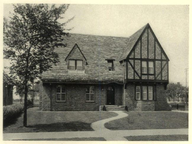
A BRICK HOUSE WITH WOOD SHINGLES. INTERIOR WALLS ARE CONSTRUCTED OF WOOD STUDS FINISHED IN PLASTER. FLOORS ARE OF WOOD. TRIM, DOORS AND WINDOWS ARE ALSO OF WOOD. THE HOUSE IS HEATED BY VAPOR AND OIL AND HAS A SEWER SYSTEM OF DRAINAGE AND PUBLIC WATER SUPPLY. ELECTRICITY IS INSTALLED. THE BUILDING WAS ERECTED IN 1925 AT A COST OF 55 CENTS PER CUBIC FOOT
