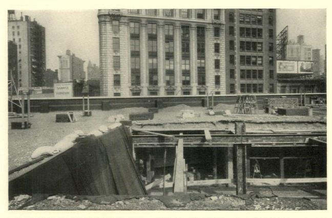
ROOF OF COLONNADE BUILDING SHOWING COURT OPENED FOR CONSTRUCTION. NOTE WATERPROOF BOXES OVER COLUMN STUBS TO PROTECT LOWER STORIES FROM THE WEATHER
