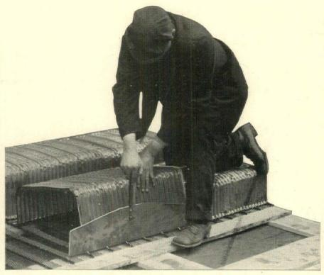
Truscon Floretyles are sprung into prongs in the Locktvle Lath. A fast, labor-saving type of construction.
