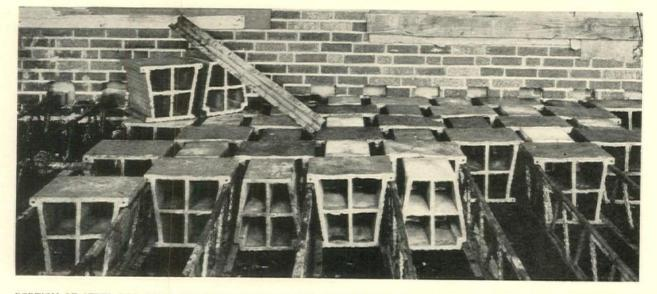
PORTION OF STEEL BAR JOIST AND HOLLOW TILE FLOOR CONSTRUCTION SHOWING THE ALTERNATING "A" AND "B" TILE AND THE METAL SHOE USED TO HOLD THE "B" TILE AND CONCRETE UNDER THE JOISTS. THE "A" TILE ARE SUPPORTED ON THE JOISTS BY MEANS OF LUGS OR FLANGES FORMED ON THE TOP. THE BOTTOM FLANGES OF THE "A" TILE SUPPORT THE METAL SHOE
