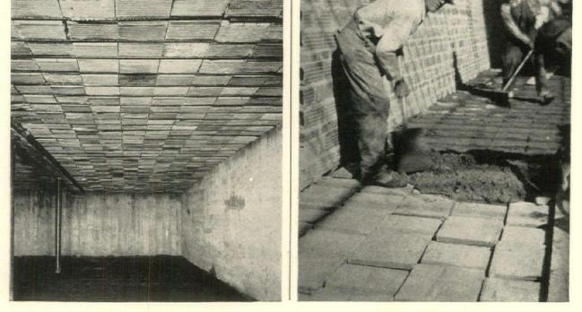
AT LEFT: UNDER SIDE OF STEEL JOIST AND TILE FORMLESS FLOOR CONSTRUCTION USED IN A BUILDING AT LORAIN, OHIO. AT RIGHT: PLACING CONCRETE BETWEEN JOISTS AND OVER HOLLOW TILE FLOOR ARCH
