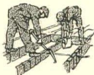
Grouting ceiling slabs
