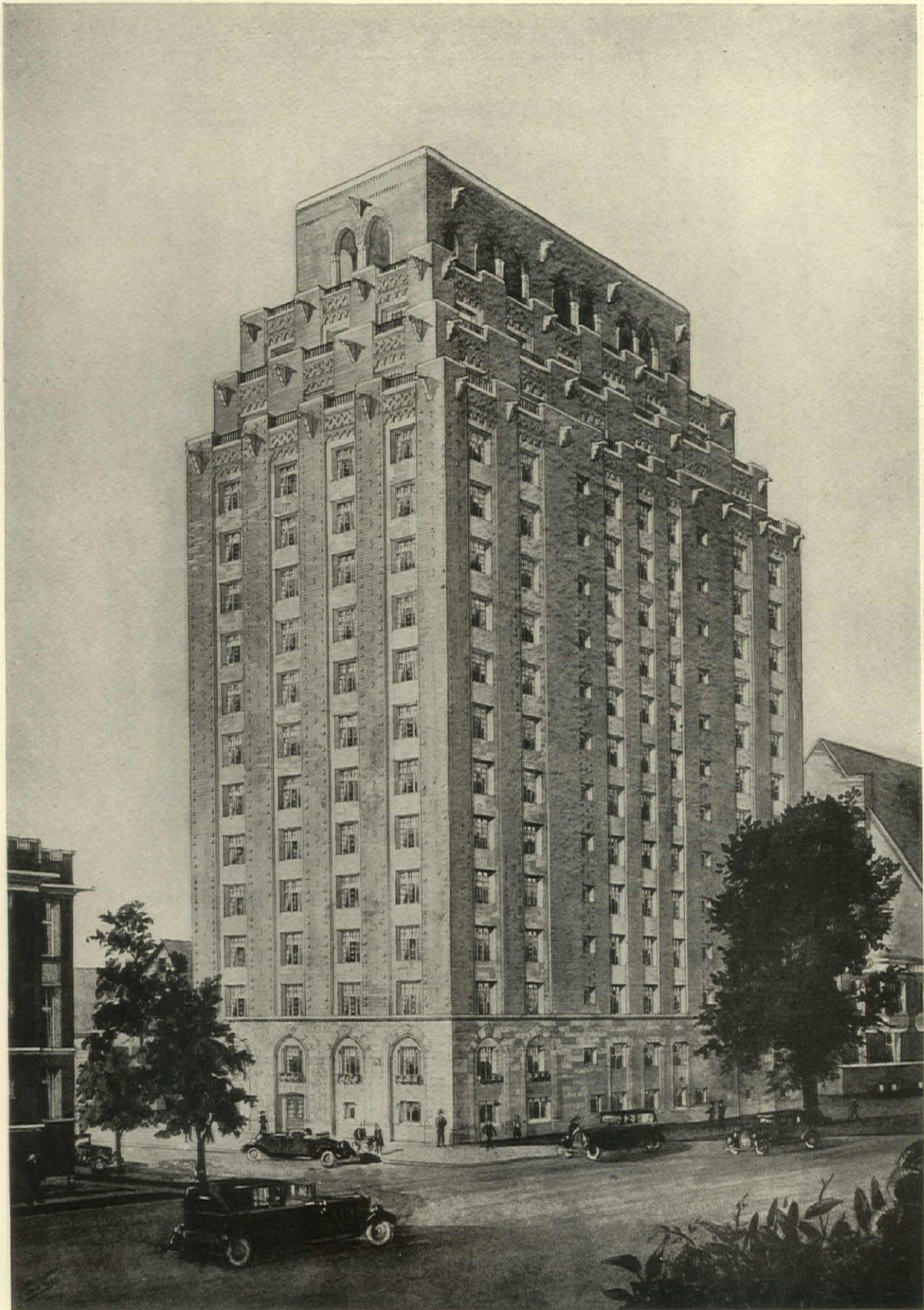
APARTMENT HOUSE, HARPER AVENUE, CHICAGO, ILL HUSZAGH AND HILL, ARCHITECTS
