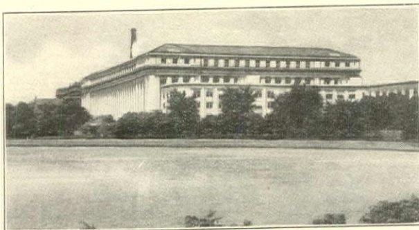
U. S. BUREAU OF ENGRAVING AND PRINTING Hot Water Supplied by a Whitlock Heater
