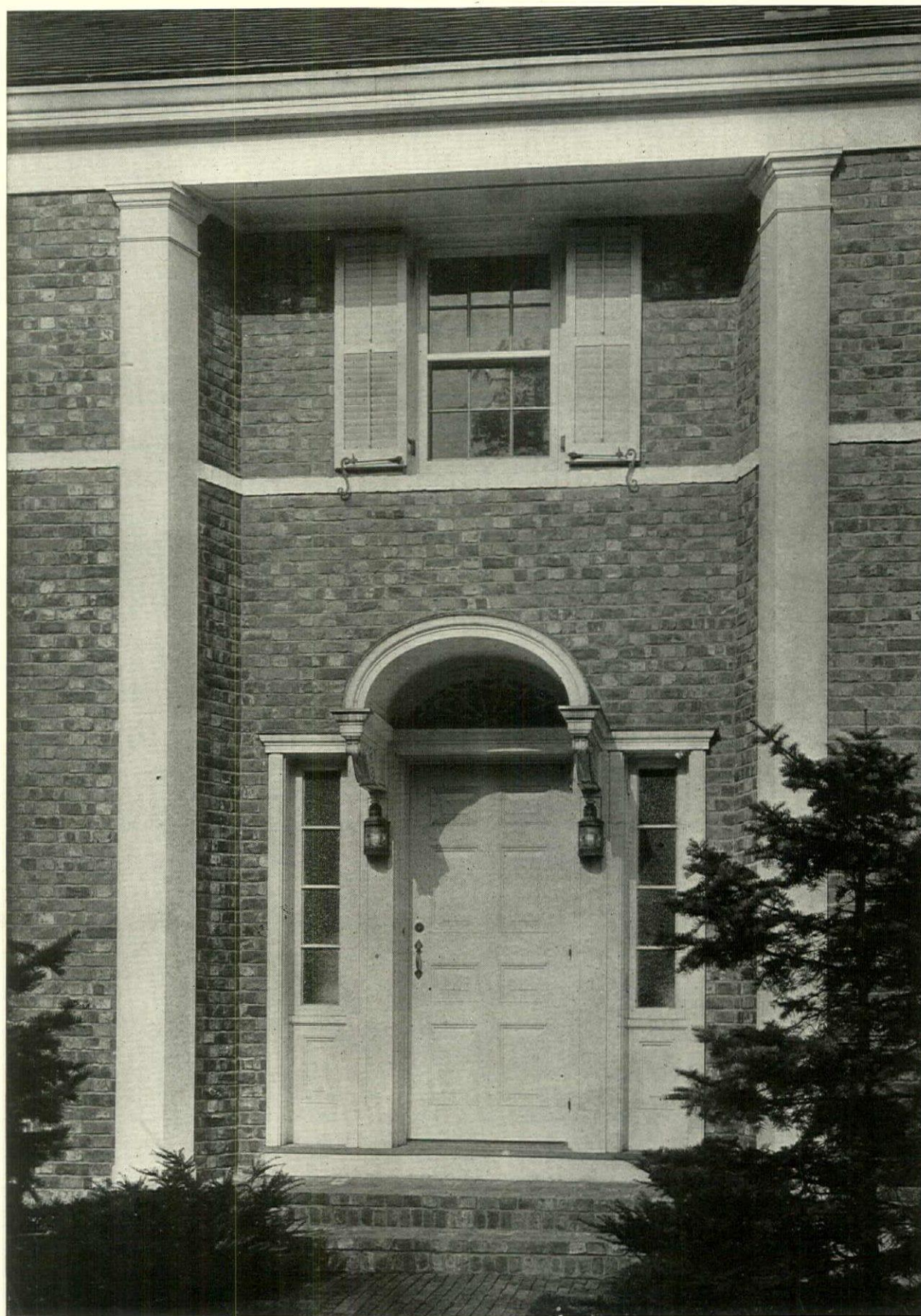
THE LOUIS WENIGER HOUSE FOR PAYNE WHITNEY, MANHASSET, LONG ISLAND, N. Y. LA FARGE, WARREN & CLARK, ARCHITECTS
