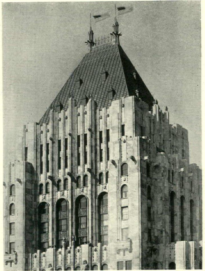
A roof of mottled green terra cotta is combined with ceramic gold in a manner which is in pleasing contrast to the marble walls below. The Fisher Building, Detroit, Michigan. Albert Kahn, Inc., architects and engineers
