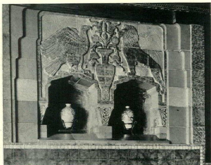
Low-relief overmantel panel above a tile fireplace, as unusual in character as in the use of terra cotta for this purpose. Community House, New York City. Henry B. Hertz, architect
