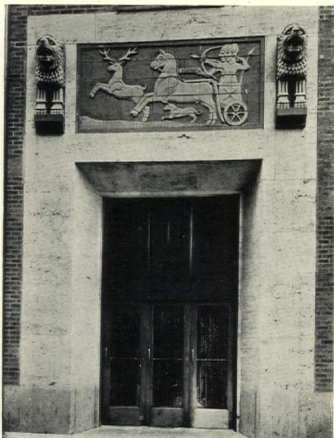
Conventional lions and a polychrome panel are used as inserts in an unusual combination with Travertine in a loft building at 130 West 30th Street, New York City. Cass Gilbert, architect
