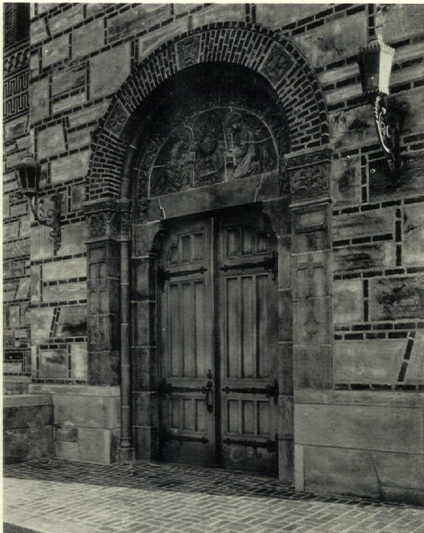
A frank and effective handling of terra cotta jointing around the doorway is typical of the requirements of the material. Terra cotta has been intelligently used for both the interior and exterior of the Chapel of St. Catherine, St. Paul, Minn. H. A. Sultwold, architect
