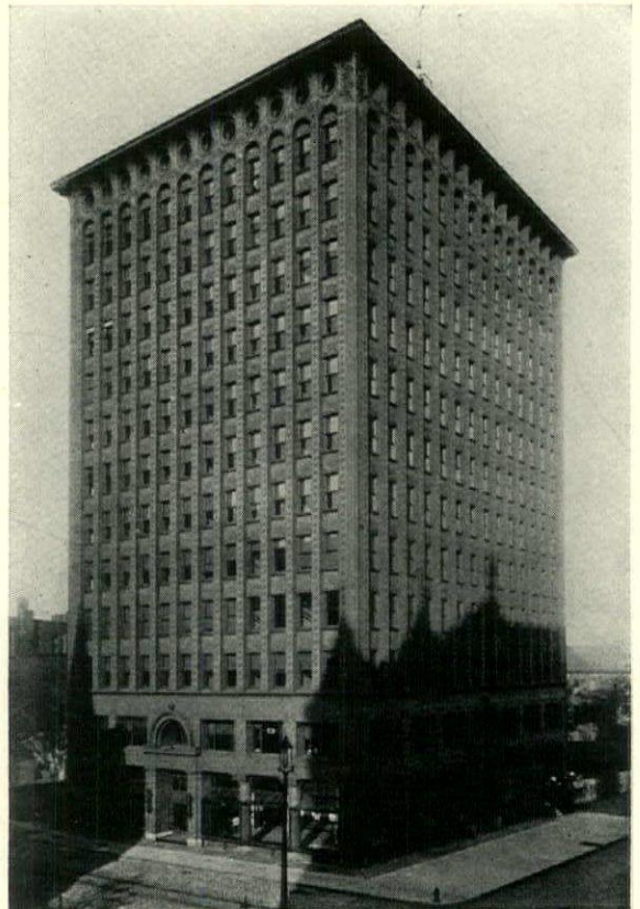
Principles upon which Louis Sullivan based his designs are seen in the Guaranty Building, built in Buffalo, New York, about 1895
