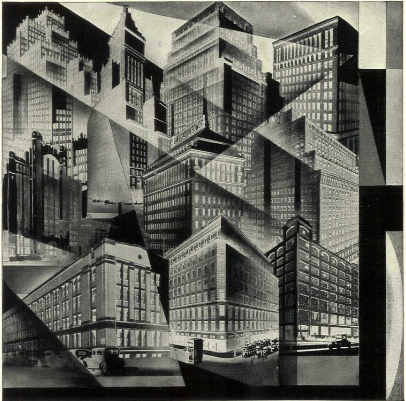
Southwestern Bell Telephone Co. Building St. Louis, Missouri
