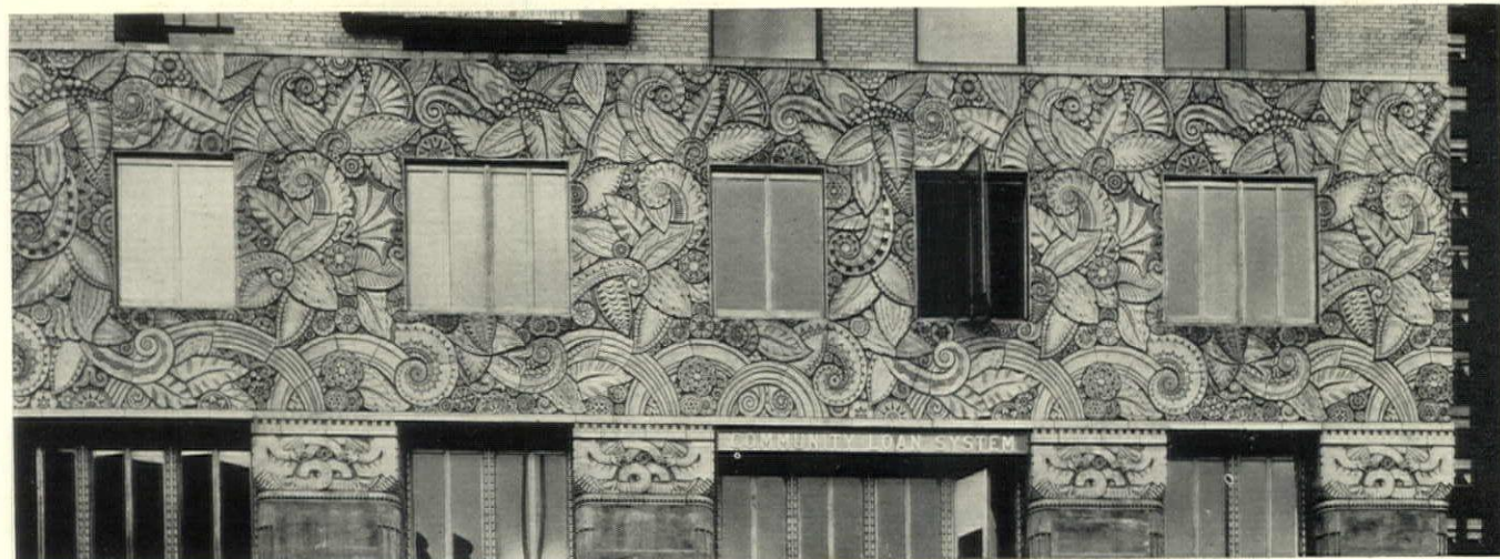
An excellent example of delicate yet bold incised low-relief modeling in terra cotta that has a distinctly "modern" flavor. This band, which extends around the fourth story of the Chanin Building, New York City, is about ten feet high, and its details are easily visible from the street. Sloan & Robertson, architects
