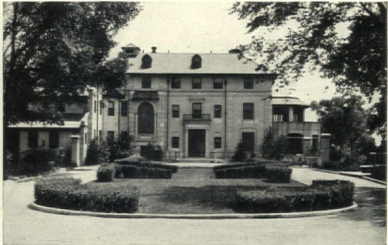
Seventeen telephone outlets provide for complete telephone convenience in the residence and garage of Mr. Edward Schmidt, 16960 East Jefferson Avenue, Detroit. The telephone wiring is carried in conduit built into the walls and floors. RAYMOND CAREY, Architect, Detroit, Michigan.
