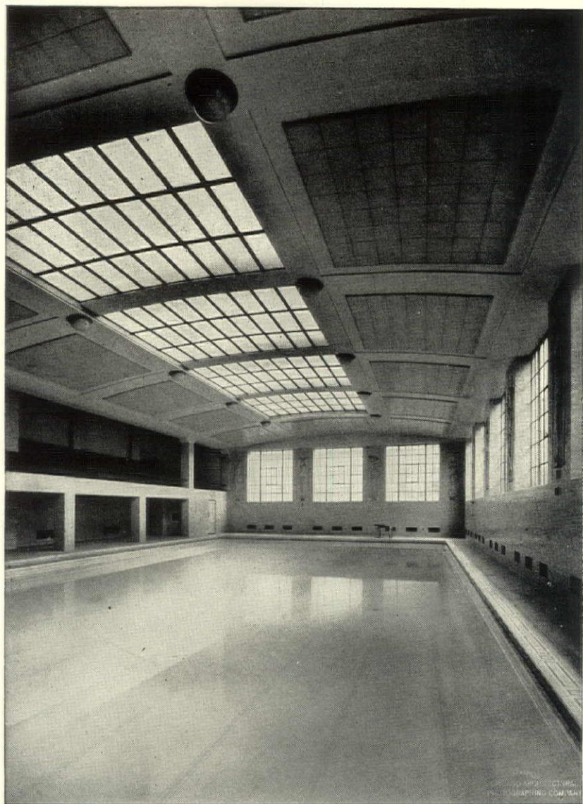
Johns-Manville Sanacoustic Tiles installed as ceiling of Girls' Swimming Pool, Oak Park and River Forest Township High School, Oak Park, Ill. Childs & Smith, Architects, Chicago, Ill.
