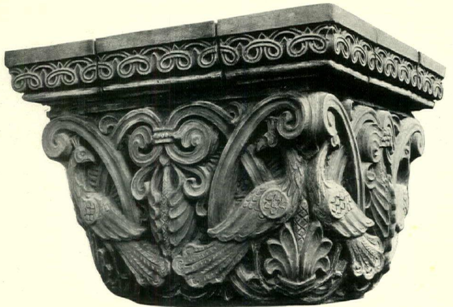
Well modeled capital that shows a sympathetic handling of burned clay. The design "flows" and "hangs together" most pleasingly. The background is neutral bluish green with raised surfaces of soft mottled color. Chapel of St. Catherine, St. Paul, Minn. H. A. Sullwold, architect
