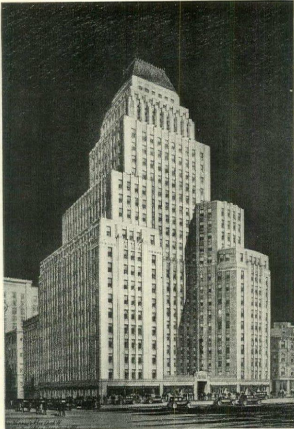
Structural corners were necessary for stability in masonry construction, but are no longer required and need not be expressed in the veneer
