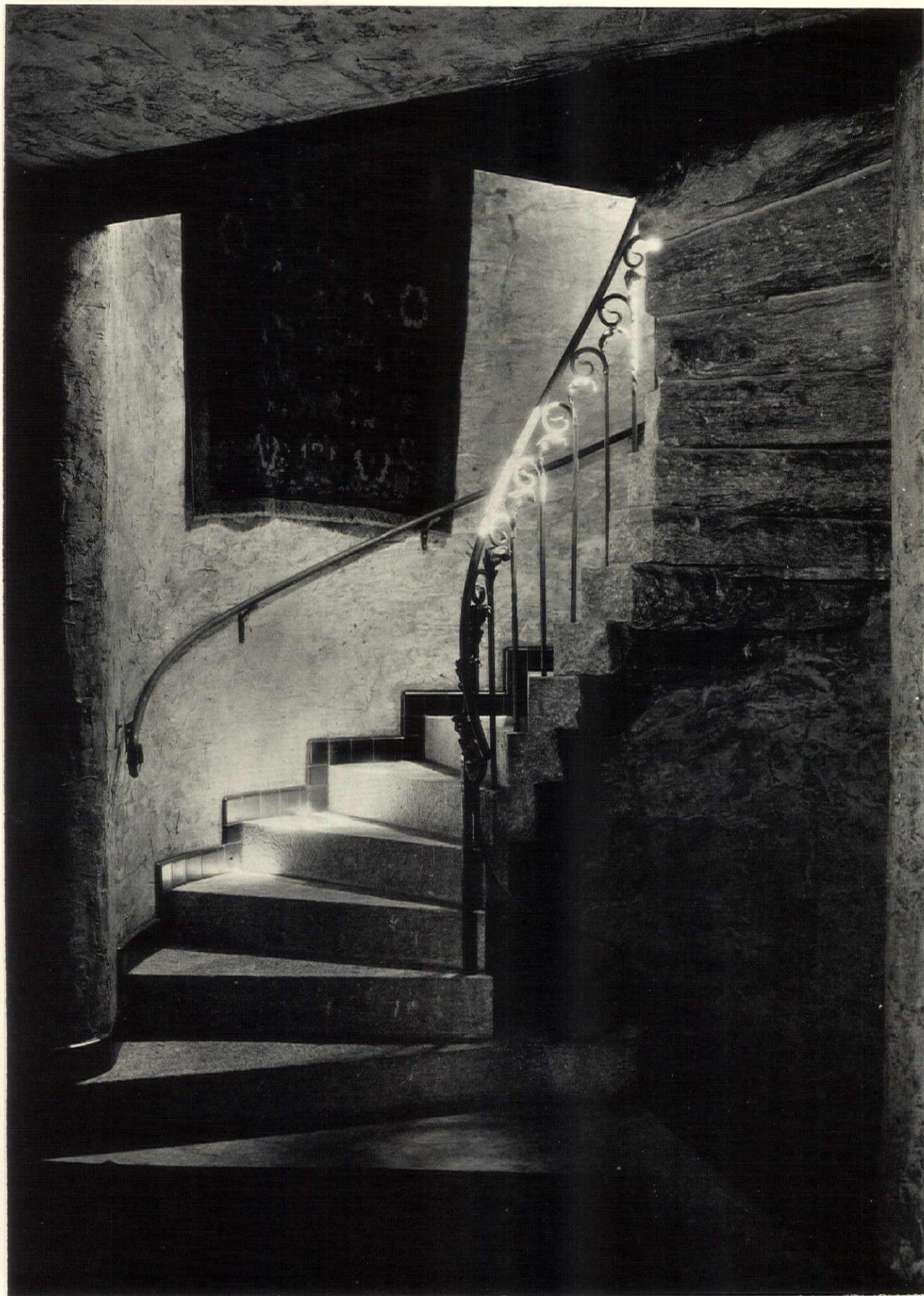
There is a medieval atmosphere about the tower stairs that is at once apparent. The steps are of local stone cut on the job by native craftsmen. The wrought iron hand rail, tile stair string and rough plastered walls have a definite relation that satisfies the eye. William Waldo Dodge, Jr., architect
