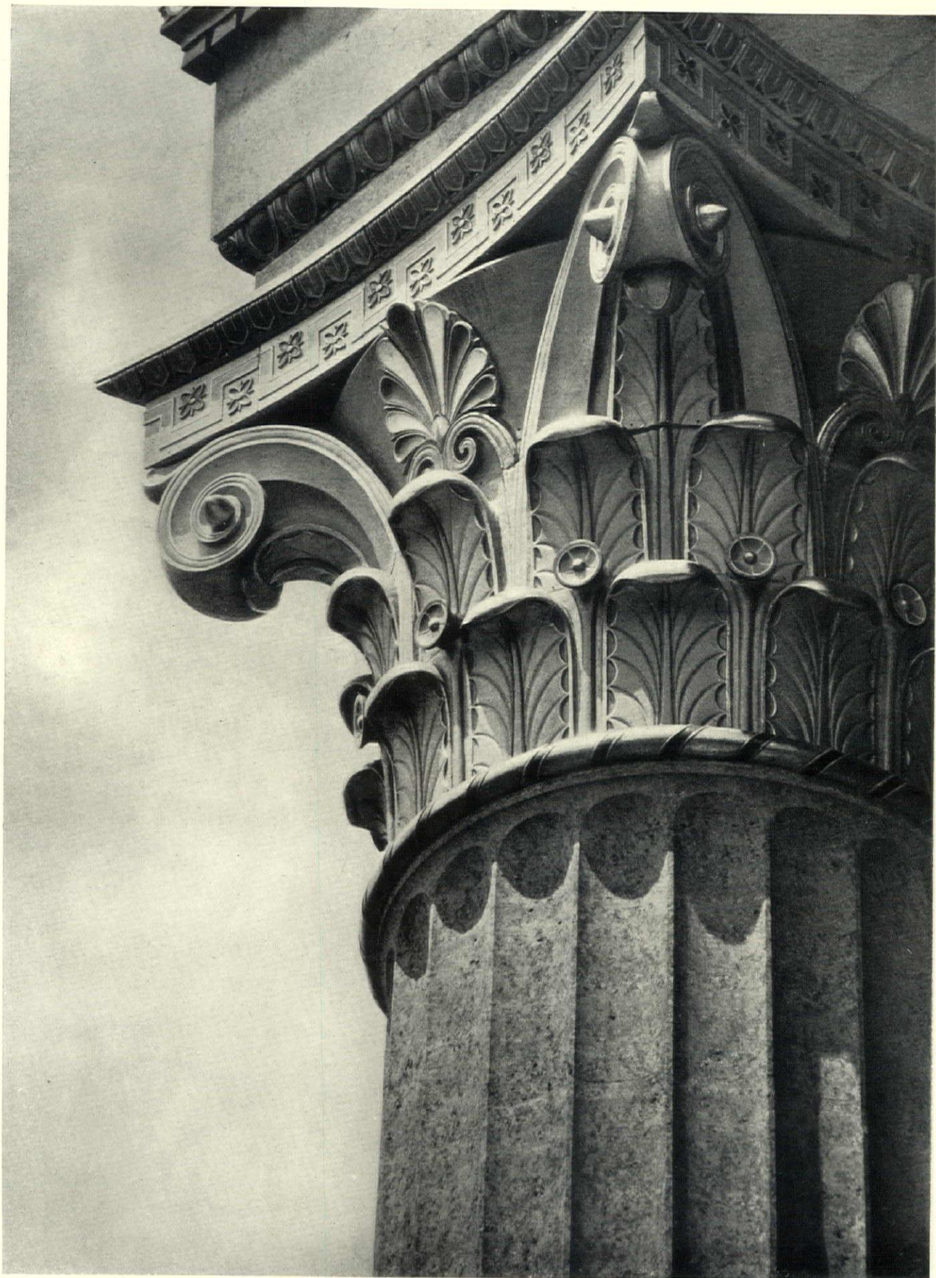
B RILLIANT polychrome terra cotta capital of the portico of the Philadelphia Museum of Art. Note the modeling of details to define color areas, which are largely gold, scarlet, vermilion and tan. The cap is 5'-2" in diameter at the neck, 6'-2" high and 7'-0" wide over all. Horace Trumbauer, C. C. Zantlinger & C. L. Borie, Jr., associate architects
