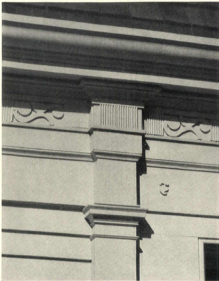
Cornice detail in Colonial tradition from the house of Allan McDowell, Kent, Conn. Designed by Chas. Wellington Walker, architect
