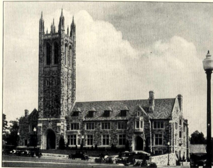
MEMORIAL MUNICIPAL BUILDING, NORWOOD, MASS. WM. G. UPHAM, ARCHITECT
