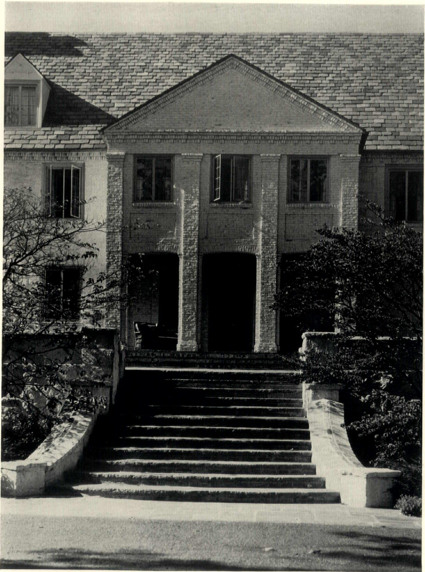
Reminiscent of early American architecture in composition, this house designed by Julius Gregory has a distinctly modern flavor in its details that is refreshing, rational and individual
