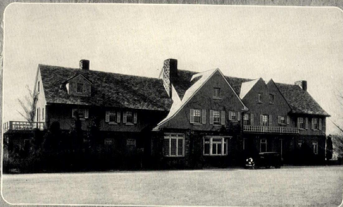
Residence at Rye, New York, Reroofed with Tudor Stone Henry Toombs, Architect for renovations
