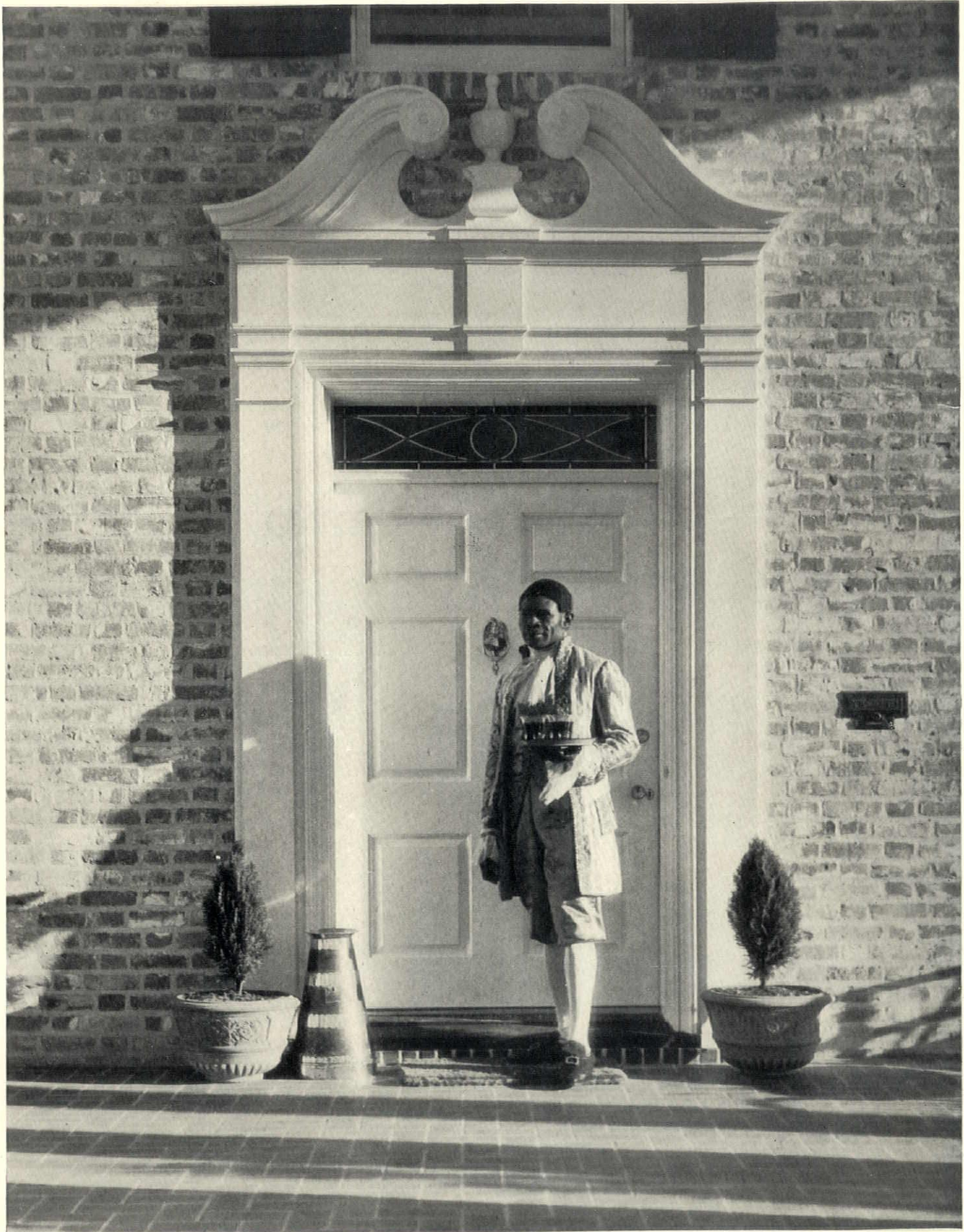
Refinement in mouldings, combined in a dignified composition, offers a pleasing contrast in color, texture, and scale to rough brick. The above doorway of Georgian inspiration in the entrance of the T. J. Bettes house, Houston, Texas; Charles W. Oliver, architect
