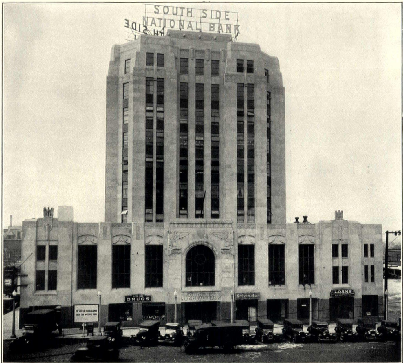
South Side National Bank, St. Louis, Mo. St. Louis Bank Bldg. and Equipment Co., Architects. Fruin-Colnon Contracting Co., Builders. Built of Gray Indiana Limestone.
