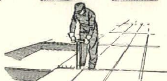
Tying the reinforcement
