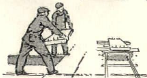
Laying a Gypsteel slab
