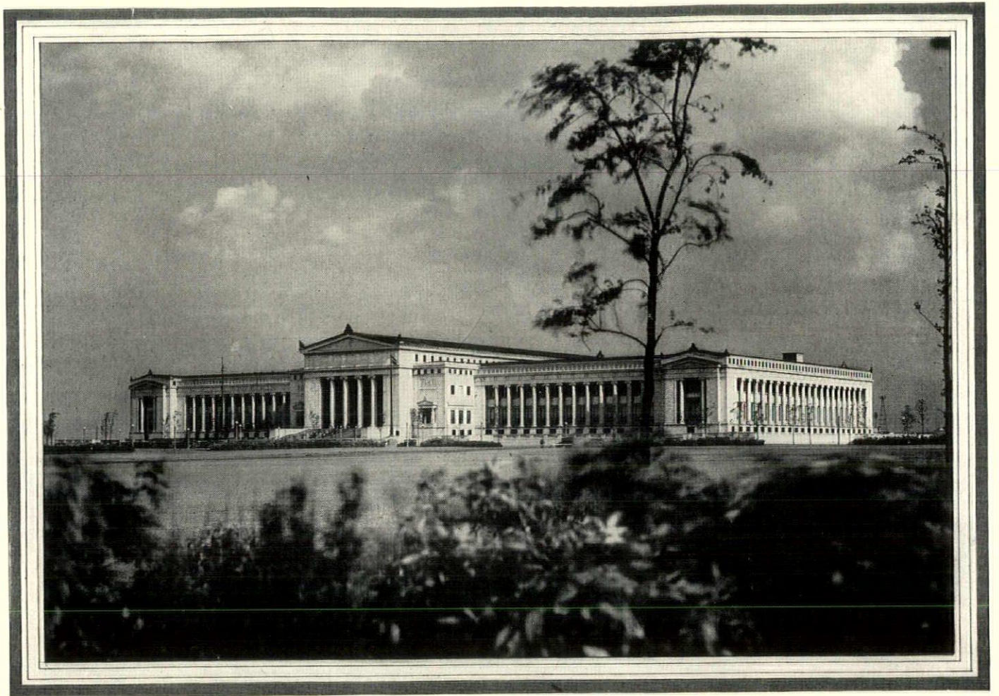
FIELD MUSEUM, CHICAGO, ILLINOIS GRAHAM, ANDERSON, PROBST AND WHITE, ARCHITECTS
