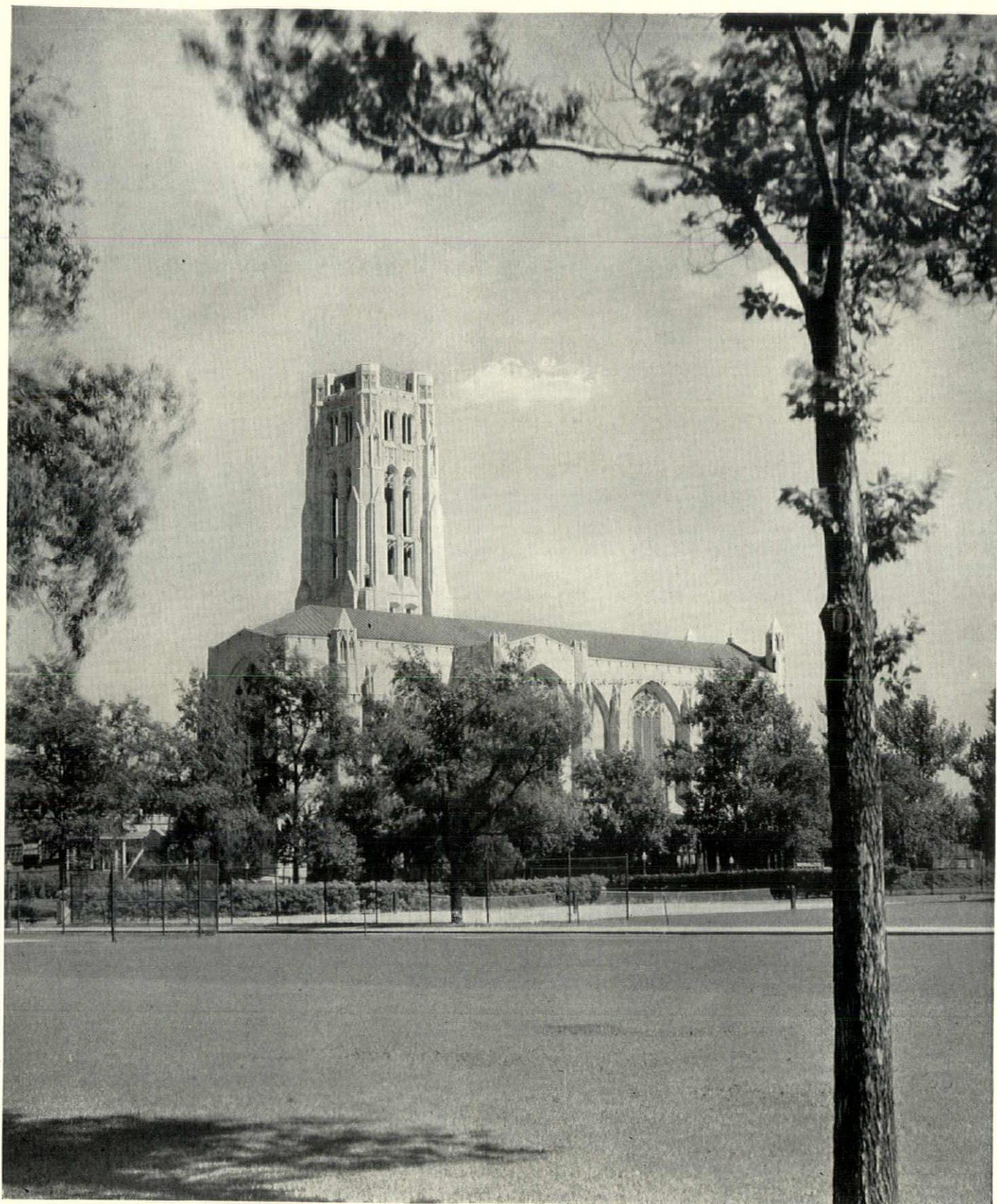
The new University of Chicago chapel, considered by many architects as one of the finest examples of modern Gothic architecture in America, was among the last achievements of the late Bertram Grosvenor Goodhue. Roof of Federal cement tile made with Universal portland cement. Leonard Construction Company, contractor; Universal cement furnished by Consumers Co., both of Chicago.
