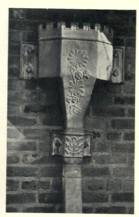
GUTTER, LEADER HEAD, and cistern combined in an unusual manner. The composition is not obtrusive due to the quality of self effacement that is more or less characteristic of lead. The raised design noticeable on the cistern is used with restraint on the leader head and omitted on the gutter. The serrated edge of the head is recalled on the gutter. This example is from the gardener's cottage of the Holmes Estate, Sands Point, N. Y. Edgar Williams, architect
