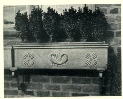
FLOWER BOXES OF LEAD are practical as well as ornamental. Lead is susceptible to a wide variety of uses. When exposed to the atmosphere, a suboxide or tarnish is formed on the surface by the union of oxygen of the air with the lead. If the tarnish is not removed it protects the lead against further oxidation
