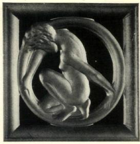
Perforated ventilating grille of moulded glass designed by Frederick Carder. The units are about eight inches square
