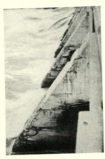
How excess water causes disintegration. From "Basic Principles of Concrete Making"
