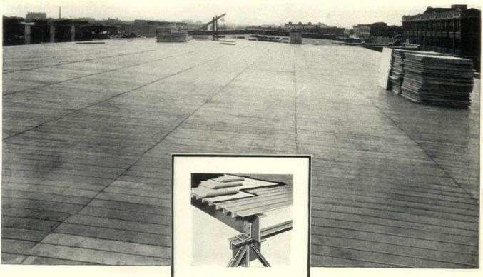
N PERMANENT roof construction, weight is the cost determining factor. When light weight is combined with firesafety and permanence in a material requiring absolutely no maintenance, you have unquestionably the most economical permanent roof obtainable.
