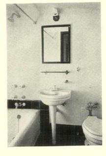
The lavatory was designed by Kenneth Murchison as a space-saving unit. It has a narrow rim with dimensions from front to back that are less than usual
