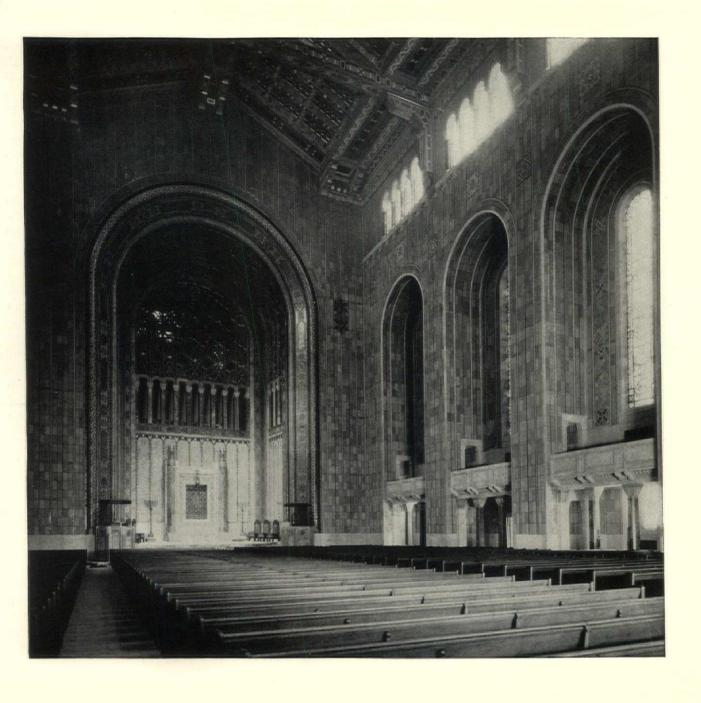
A SIDEWALL INSTALLATION OF AKOUSTOLITH SOUND-ABSORBING STONE IN TEMPLE EMANU-EL, NEW YORK CITY, IN A GRADATION OF COLOR FROM LIGHT AT THE BASE TO DARK AT THE CEILING AND WITH GOLD CERAMIC INSERTS.
