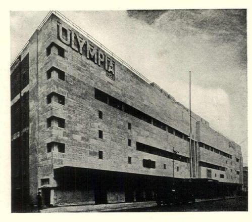
EMPIRE HALL, Olympia, London, is the first multi-storied exhibition building to be erected in England. The horizontal treatment of the facade provides permanent fittings for advertisements of the various exhibitions. The marquise is equipped with reflectors for flood lighting the exterior. From "The Architects' Journal," for January 29, 1930
