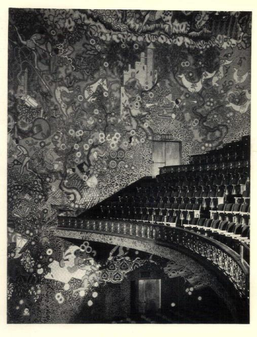
EGG SHAPED IN PLAN and section, the walls and ceiling of the Ziegfeld Theatre reflected sound waves into numerous centers, and resulted in defective acoustics. At the right are shown the plans of the orchestra and balcony floors
