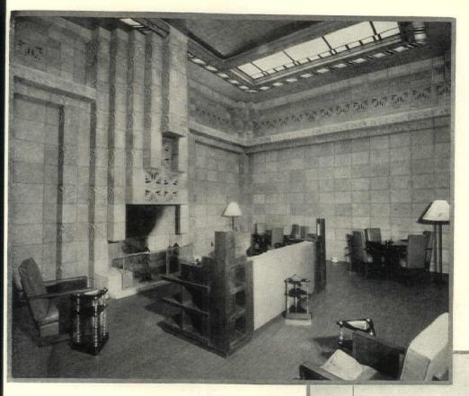
To the left, an inviting corner in the smoking room of Arizona-Biltmore Hotel, Phoenix, Arizona. Below, the unique exterior. Built of reinforced concrete, faced with cast stone blocks. Interior walls also of cast stone, in plain and conventional designs. Albert Chase McArthur, Phoenix, Architect; Frank Lloyd Wright, Associate; S. M. Benet & Co., Beverly Hills, California, Contractors.
