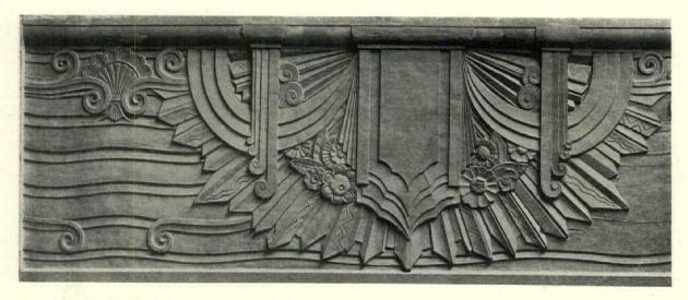
Model for a plaster frieze that indicates the tendency in the design of modern ornament to make use of flat and beveled surfaces to obtain interesting light reflecting areas
