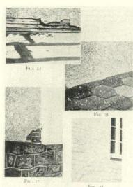
Fig. 23 Staces is absorbent and chould be kept fix inches above flat, watered incluser. Fig. 26 Pobbles used for a poblic-dash fluid bound be firmly imbedded in the staces. Fig. 27 Wooden strips at the bottom of a staces wall present water from destining off. Fig. 28 Poor workmanship dischared by the outlining of the brick through the staces.
