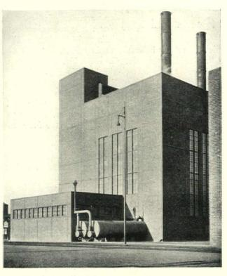
The wide expanse of brick wall surfaces are broken by a pattern of horizontal and vertical lines and effectively placed and proportioned fenestration in the central coking plant of the gas works at Nordstern. The main boiler house is shown above. From the April, 1930, issue of "Baukunst"
