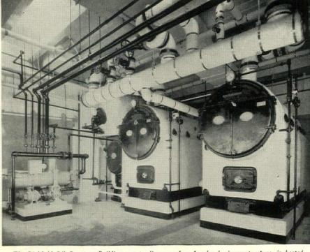
The Richfield Oil Company Building, outstanding new Los Angeles business structure, is heated by three Pacific Welded Steel Boilers burning oil. Architects, Morgan, Walls & Clements. Mechanical Engineer, Ralph E. Phillips. Heating Contractor, Thomas Haverty.
