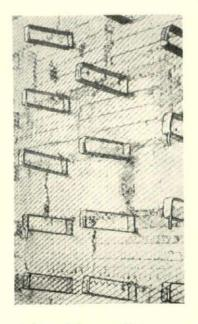
The Red Top Innerwall Furring Bracket, introduced by the United States Gypsum Company, 300 West Adams Street, Chicago, offers a practical method of furring metal lath over all types of masonry walls. These brackets are set in the soft mortar joints as the work progresses. The brackets have prongs which serve to fasten the metal lath. Furring may be from 11/4" to 41/4" in depth. providing a dead air space which can be used for electrical con-
