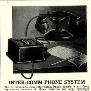
The Stromberg-Carlson Inter-Comm-Phone System is satisfying the service demands of offices, factories, and large residences where simultaneous conversations are necesary, but where the volume of traffic is not large enough for a switchboard system and a paid operator.
