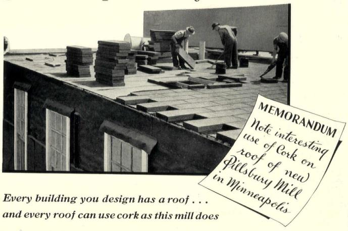
I N a flour mill, the roof must do more than just shed water. In every building, a really good roof stops heat almost as completely as it shuts out rain.
