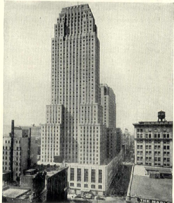
The Carew Tower Building, Cincinnati, Ohio, W. W. Ahlschlager, Architect, Starrett Brothers, Inc., Builders. One of Cincinnati's largest office buildings, housing a hotel of 732 rooms, and a garage with lobby entrances also lined with Atlantic Wall Units.
