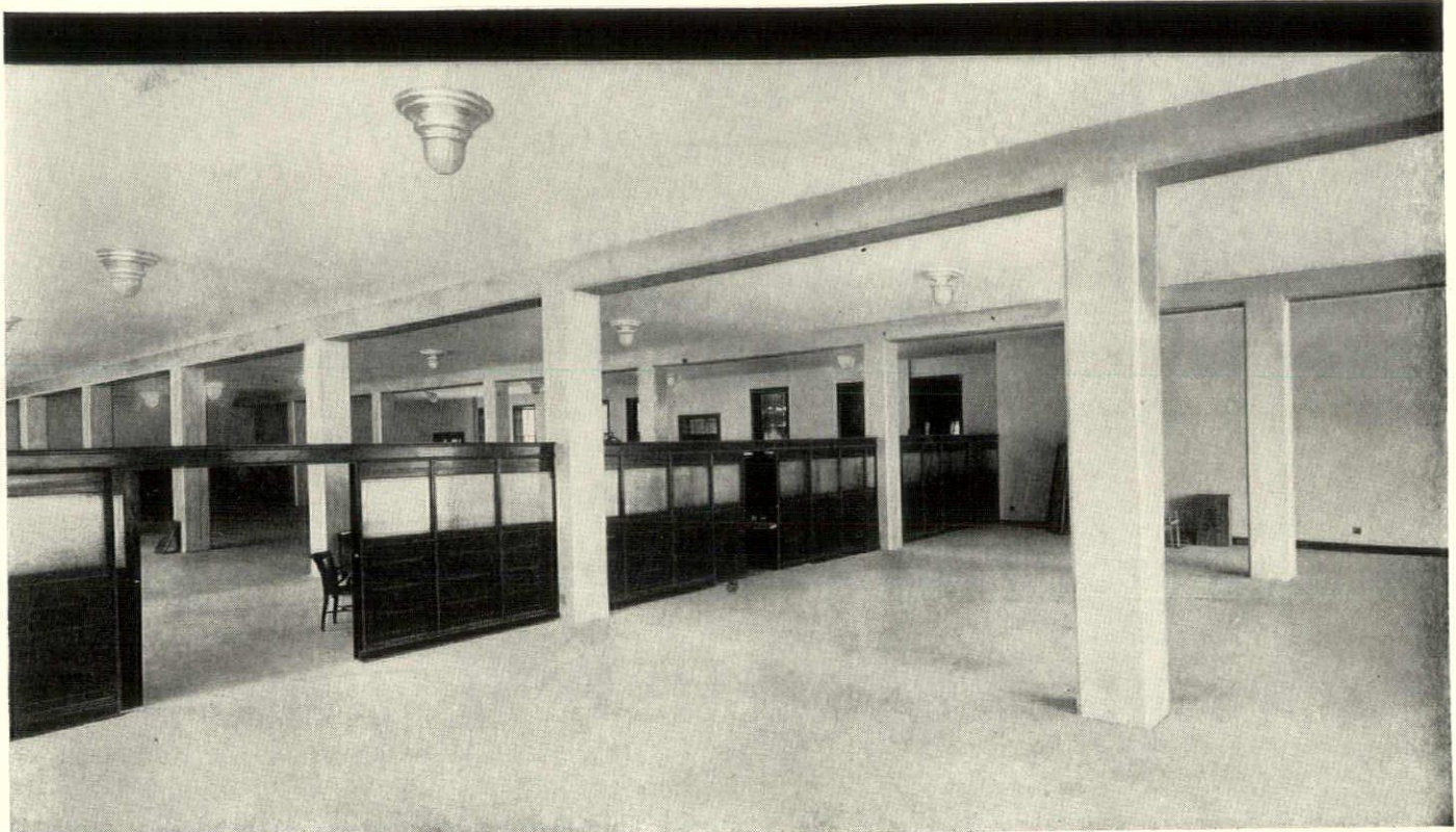
Concrete columns and floors at the newly remodeled Saddle & Sirloin Club, Chicago; high-early-strength concrete made with Universal Atlas methods and cement used in the construction. Poirot Construction Co., Chicago, contractor.
