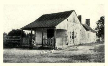
First of logs, then plastered over, and finally shingled
