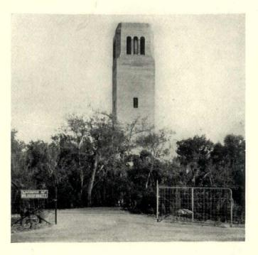
OF ROUGH CAST CONCRETE, the campanile tower on the estate of George P. Brett, Miami, Florida. The structure is eighty feet high and sixteen feet square; it is designed to resist a storm of hurricane velocity. A water tank is at the top. Wade & Oemler, architects
