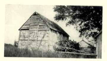
Half timber and stone nogging with wide joints of white mortar
