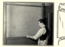
First putty is palmed into the grooves, then it takes only a moment to slide the giass into position.
