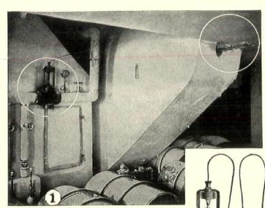
A No. 942 Sylphon Temperature Regulator on air conditioning equipment in a large candy factory.
