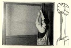
After the glass is inserted, a simple downward pull on the telescopic member retains it in place. The putty is scraped smooth, the glass is cleaned, and the job finished.
