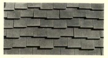
Tapered Asbestos Shingles
