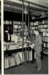
Cashier's Desk on main floor Main floor view of Sedgwick Lift used for handling books between main floor and the mezzanine. Various styles of carrier available to meet specific needs.
