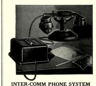
The Stromberg-Carlson Inter-Comm-Phone System is satisfying the service demands of offices, factories, and large residences where simultaneous conversations are necessary, but where the volume of traffic is not large enough for a switchboard system and a paid operator.
