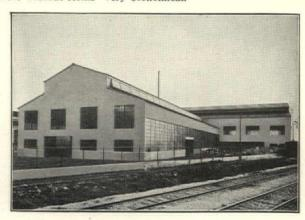
HY-RIB Concrete Sidings (built without forms)— MARK MFG. CO., Evanston, III. UNITED SASH used in all windows.
