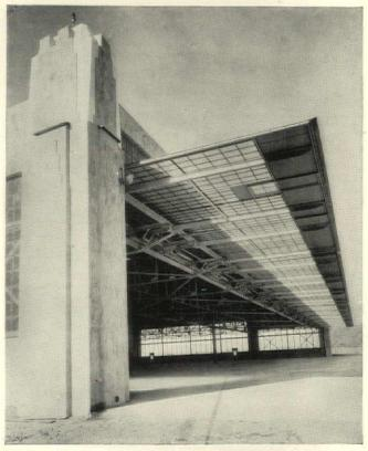
Airplane Hangar with 300-foot clear door opening. Note pass door at each end of Kanopy door.
