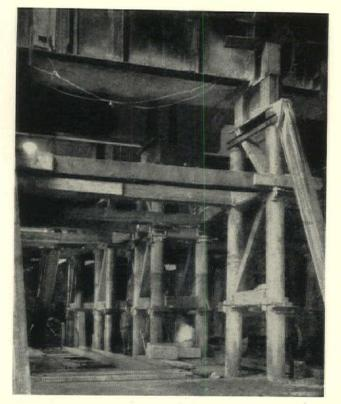
Lafayette Street subway supported on underpinning piles, showing sway bracing. From "Underpinning"
