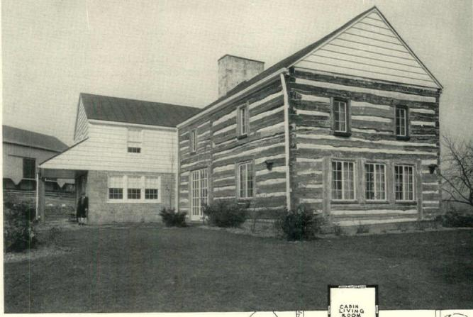
AN OLD LOG CABIN on the farm of Grant McCargo, Dorseyville, Pa., formed the nucleus of a new house. The rebuilt cabin became a living room twenty by thirty feet and two stories high. The addition is in cinder concrete block and frame. On the second floor of the new part are two bed rooms, bath and dressing room
