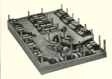
SPIRAL RAMPS FOR GARAGES. Model of saucer spiral system developed by Bishop, Knowlton & Carson, architects and engineers, and Skiles E. Test. Cars can be driven on or off ramp at any point; over 60% of cars can be parked without maneuvering. Grade about 8% at center, diameter 66'. Adaptable to buildings of various sizes and shapes, whether new or old structures
