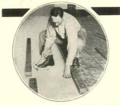
The construction principles of BLOXONEND are sound! Dovetailing the small, tough blocks endwise onto substantial baseboards and joining the built-up sections with heavy wood splines results in a degree of smoothness and durability not obtainable in other types of flooring. Write for Descriptive Folder.
