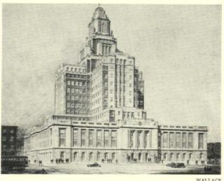
Customs House and Appraisers' Stores, Philadelphia, designed by Ritter and Shay, architects. The upper stories are cross-shaped in plan to secure maximum daylight in offices
