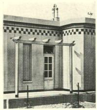
Steel houses of factory produced standard panels have been developed in France by Fillod. Various combinations of stock units, a choice of paint colors and accessory decorative elements are relied upon for individuality
