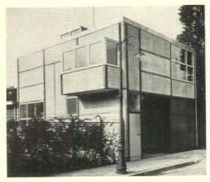
Perhaps the Dutch architect Rietveld has here forecast the future American home of enameled concrete slabs mounted in steel girders and columns
