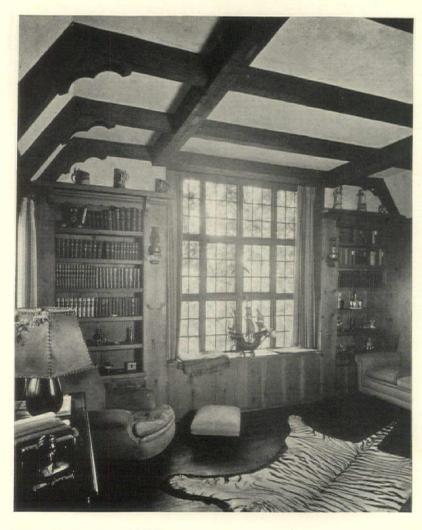
Exterior walls, brick, whitewashed. Roof, hand split cedar shakes with heavy butts stained in various shades of brown and laid irregularly. Timbers and beams, hand hewn. Porches and terrace, also entry hall floor, stone flagging in dull reds and browns. Study, at left, panelled in knotty white pine oiled and waxed to a soft satin finish. Living room, dining room and entry hall have hand hewn beamed ceilings. Living room is a story and a half high
