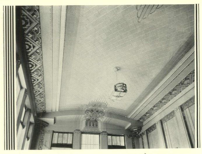
Acousti-Celotex on the ceiling of Main Banking Room, Long Beach Building & Loan Assn., Long Beach, California. Schilling & Schilling, Architects.
