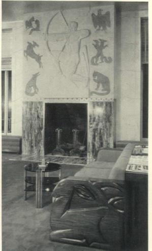
MATERIALS IN LOUNGE: Walls, parchment stretched over solid laminated panels, rabbeted at edges and blind nailed. Wall behind panels lined with galvanized iron to protect parchment from moths and vermin. Ceiling: Field, light gold leaf with ornament picked out with deep gold leaf. Ceiling fixtures have flashed opal glass panels with carved stripes. Carpet, golden brown with black border. Hangings of coarse texture running from light gold to rich brown
