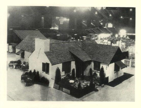
The house, built of cinder concrete blocks, was erected in four days. The cost of duplicating this house was quoted at \$4,000, complete with equipment
