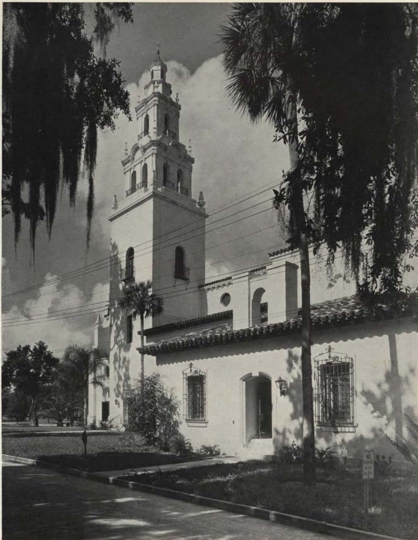
KNOWLES MEMORIAL CHAPEL ROLLINS COLLEGE, WINTER PARK, FLORIDA CRAM AND FERGUSON, ARCHITECTS; KIEHNEL AND ELLIOTT, ASSOCIATE ARCHITECTS
