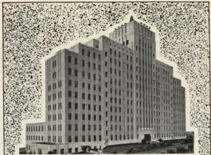
Refrigeration at the Harborview Hospital, Seattle, is supplied with Frick Carbon Dioxide Equipment
