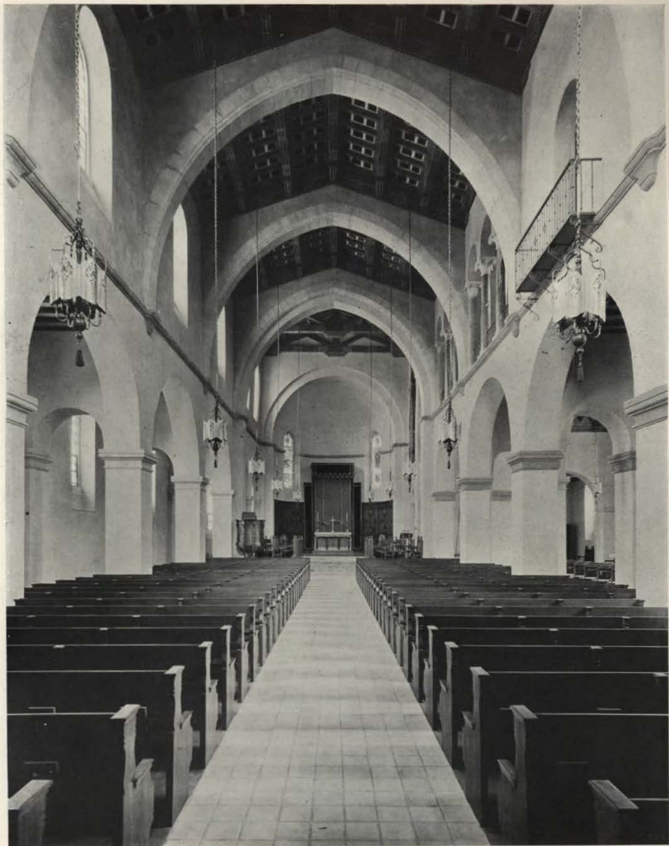
THE NAVE. Ceiling of both nave and chancel, cypress, beamed, paneled and decorated in color. Walls, plaster; arches, Florida travertine; aisle floor, unglazed red tile. Lighting fixtures, specially designed to eliminate glare, have a central baluster of wood and pierced aluminum screen about the bulbs
