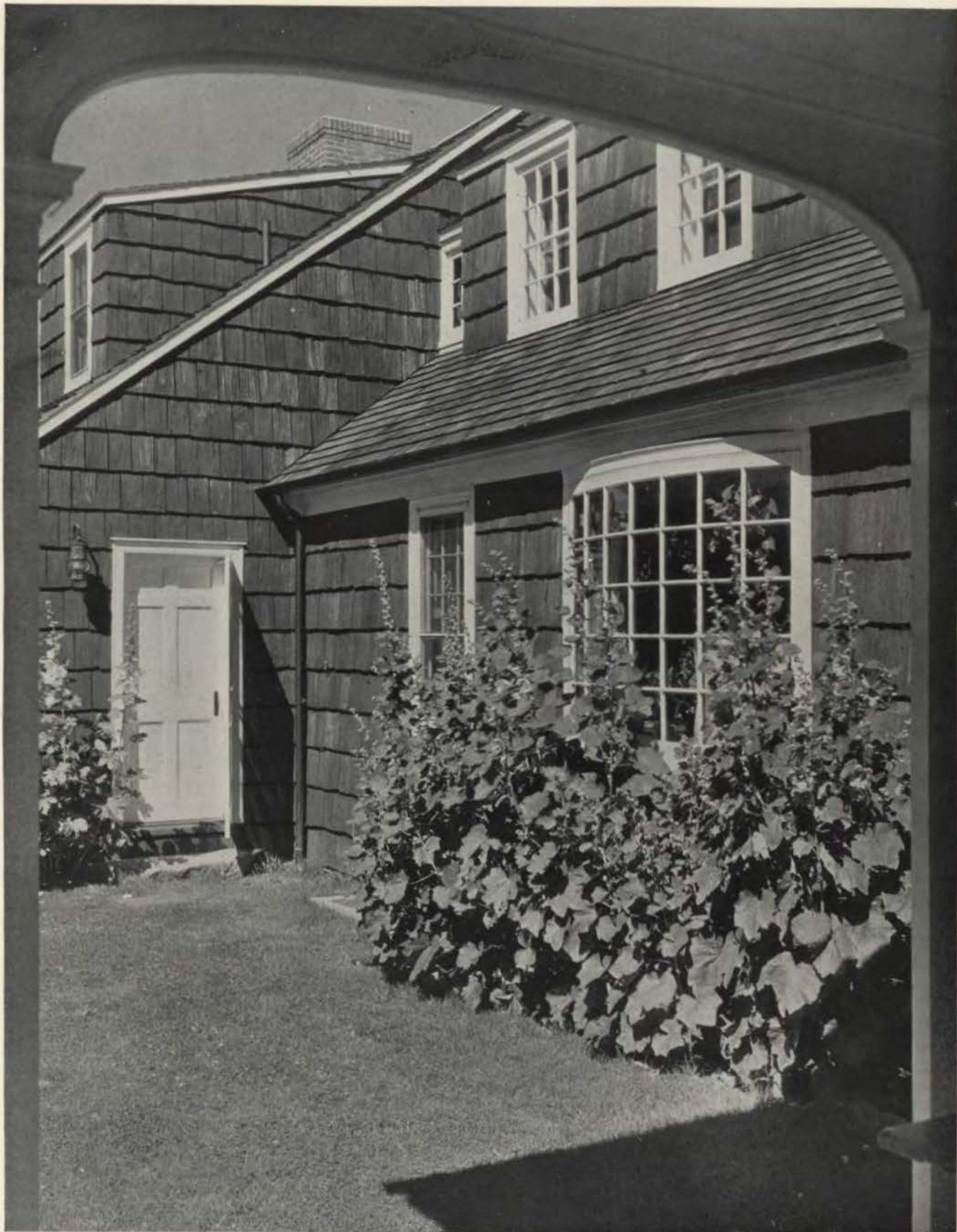
Detail of Exterior, Showing Dining Room Bay
