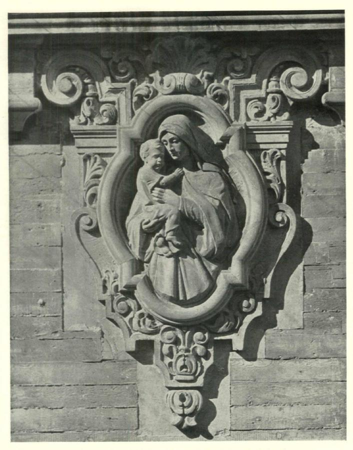
Made from a plaster of Paris mould, this plaque of concrete is integral with the wall
