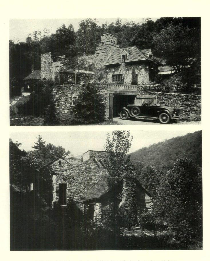
Unskilled labor built this house with native and old materials. Walls, salvaged brick and stone picked up on the site. Heavy timber framing, hand-hewn shingles, hand-forged hardware. Above: house from the drive; below, old log cabin, now used as study. Facing page, above: sun terrace; below, right, entrance detail
