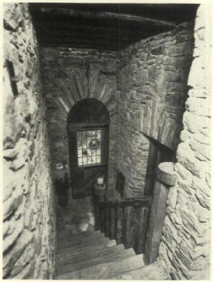
Walls and framing are solid throughout the house, most rooms being unplastered. Stonework is gray, flecked with tan, red and yellow. Brick are variegated in high colors, toned by age. Timber framing and plank sheathing are silvery gray. Above, detail of living room ceiling and gallery stair. Facing page shows main hall
