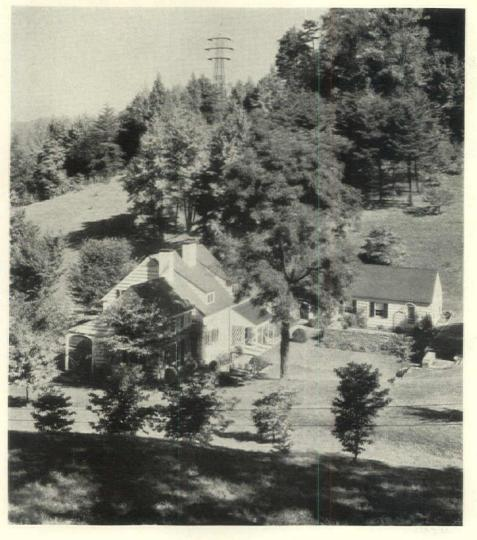
Construction: House is frame with shingled exterior painted white. Roof, shingles stained brown. Blinds painted dark green. Interior walls, plaster, painted and papered. Floors, oak, with linoleum in kitchen and baths. House contains 42,160 cu. ft. Illustrations show garden at the rear of the main house. The small building is a two-car garage that includes a chauffeur's room and bath
