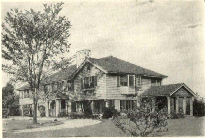
Residence at Fox Point, Wis. Furber Libby and Alfred Gillman, Architects, Milwaukee. Roof and walls stained and preserved with Cabot's Creosote Shingle and Wood Stains.
