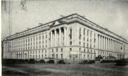
DEPARTMENT OF JUSTICE BUILDING. "Freon" air-conditioning equipment by York and Cooling and Air-Conditioning Corporation.
