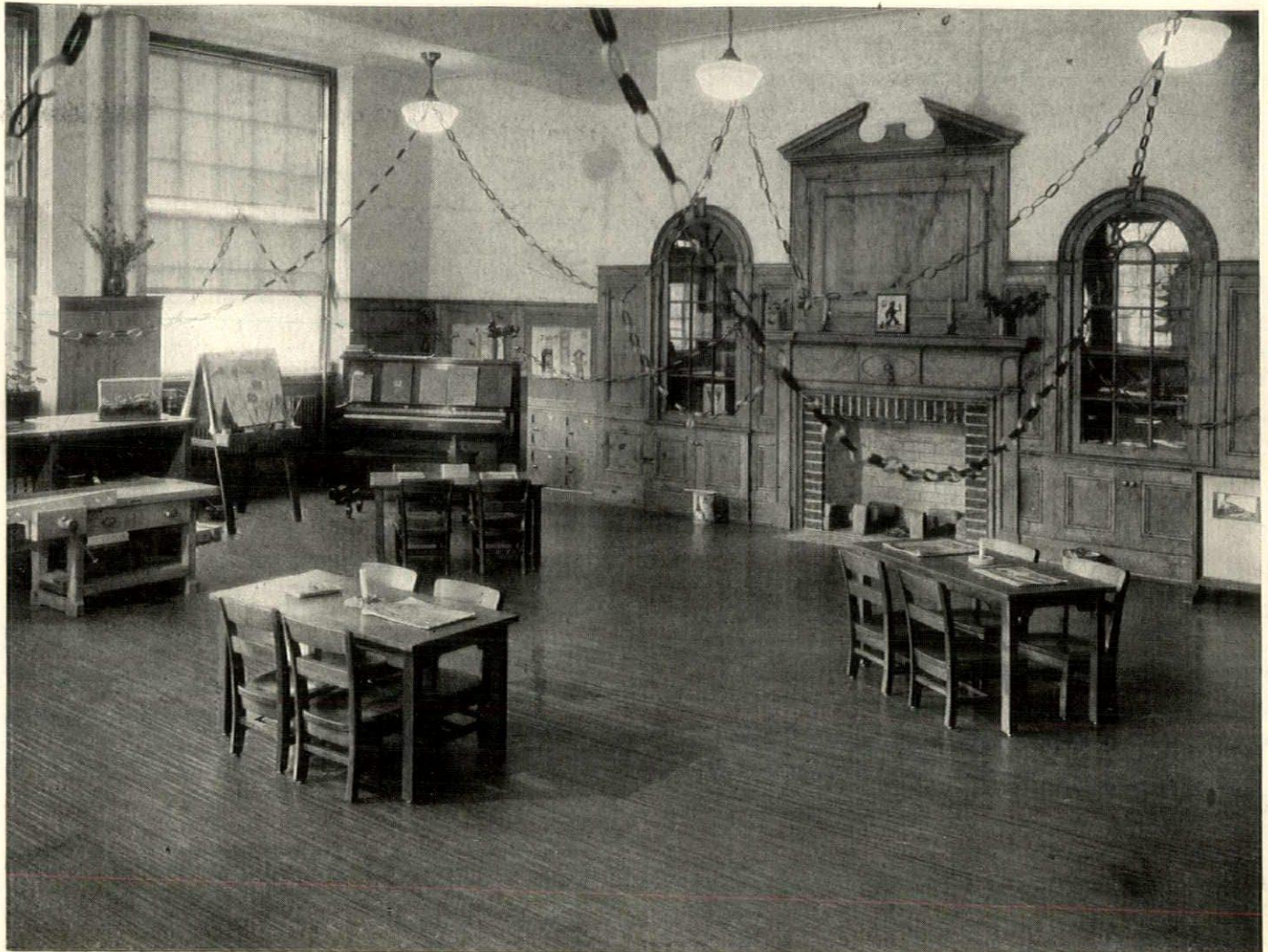
SEALEX JASPÉ LINOLEUM IN THE RIVERSIDE SCHOOL, RIVERSIDE, CONNECTICUT. Architect: WILLIAM F. DOMINICK
