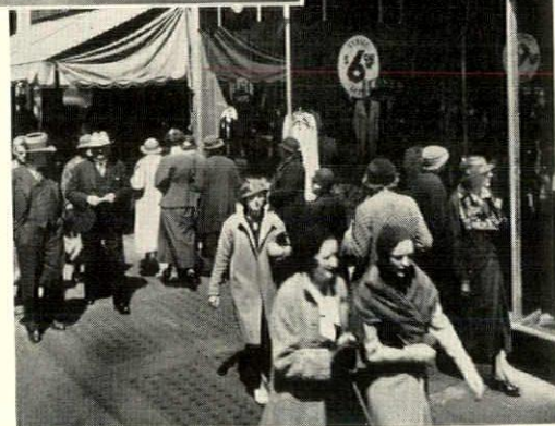
Four colors of terrazzo—all made non-slip by suitable colors of Alundum Aggregate—were used in this Lerner Store entrance in San Francisco. Installation by M. H. Gnecco & Company, San Francisco.
