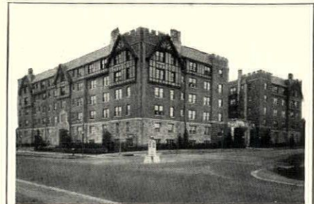
Tudor Hall Apartment In these days of high vacancies apartment owners cannot risk any heating plant failures. Where two Petro Model LA automatic oil burners are on the job, there is no such risk.
