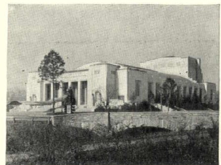
Westchester County Center The problem of heating large auditoriums presents a special set of conditions, ideally met by Petro Model LA equipment.
