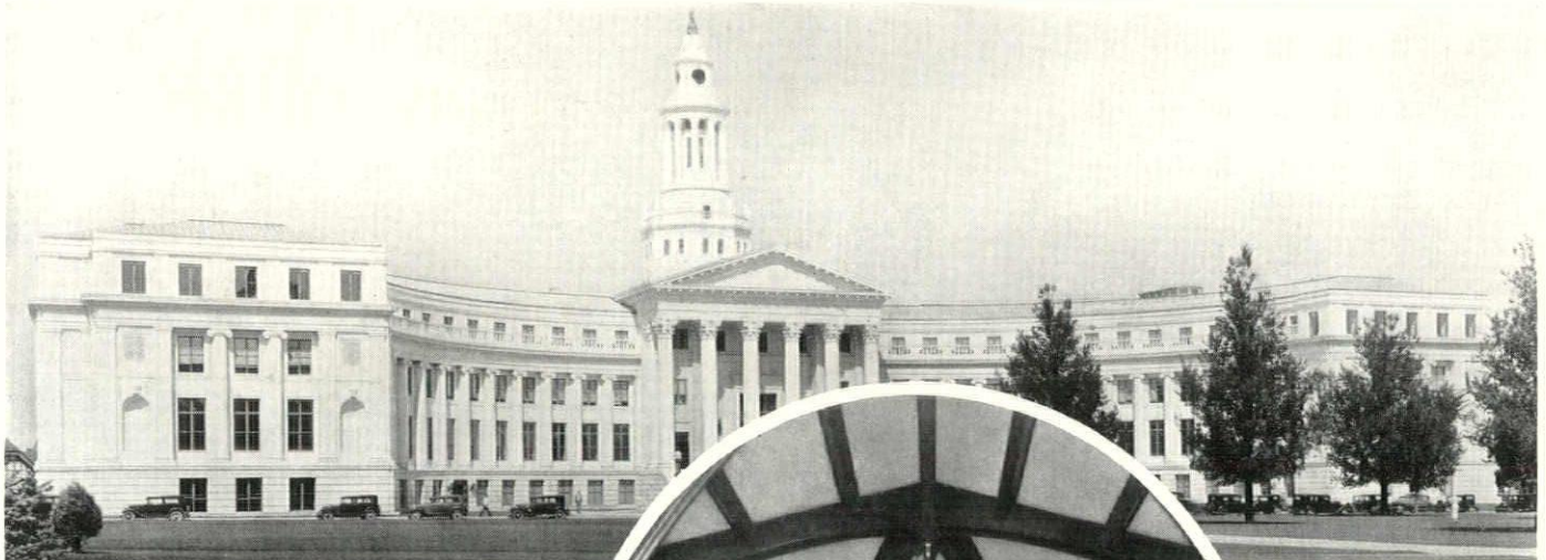
CORKBOARD —reducing expansion and contraction of steel members in the roof of the new City Hall and Court House, Denver, Colo. Shown in the illustration above.
