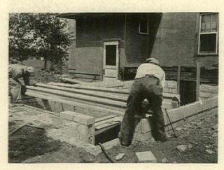
Remodeling projects using precast concrete joists claim speed and efficiency for this type of construction, and provide a fire-safe and very adaptable treatment of floors and ceilings.
