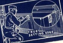
The outer edge of inner member serves as a true, unvarying line to which face of structural material is set.
