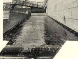
Koppers Waterproofing on sidewalk at the Pittsburgh Post Office just before final concrete course.
