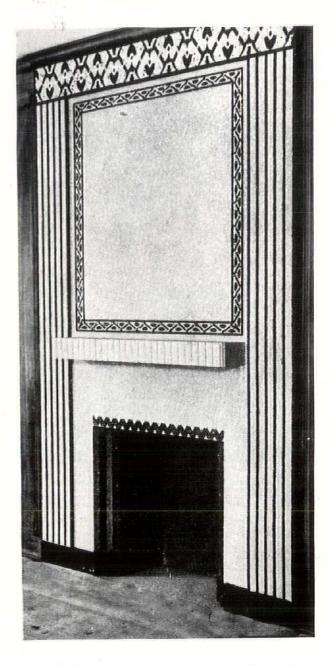
PRE-CAST CONCRETE, typified by this monolithic fireplace panel, is well adapted to use in small houses. Field, light buff ceramic aggregate; borders, red and blue; fireplace, black, outlined in red. John J. Earley, architectural sculptor
