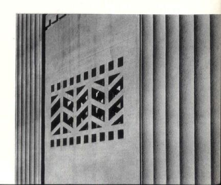
**Exposed aggregate** concrete, as the name implies, is simply concrete from which the cement paste on the surface has been removed, exposing the aggregate beneath. The two factors which determine the type of texture produced by this means are the method used in exposing the aggregate and the degree to which it is exposed. The size and nature of the aggregate itself is, of course, a factor.
