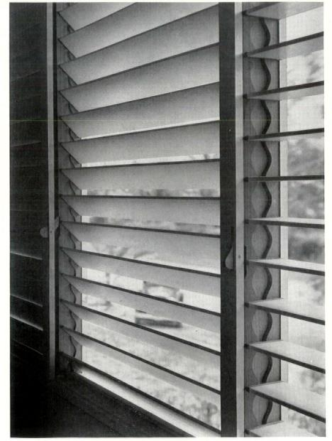
Porch shutters make possible a full utilization of outdoor living spaces regardless of weather conditions. The patented type illustrated here is much used in Nassau and the Bahamas as well as at Miami Beach. House of Galt Stockley, Office of J. and C. Skinner, architects
