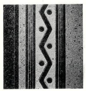
COLOR AND TEXTURE were produced in the Shrine of the Sacred Heart, Washington, D. C., by the controlled use of exposed aggregate. Main body of concrete was wire-brushed before completely set to expose the aggregate. Precast details were similarly treated after removal from plaster moulds of a type which permitted the segregation of colored particles. Murphy & Olmsted, architects: John J. Earley, architectural sculptor
