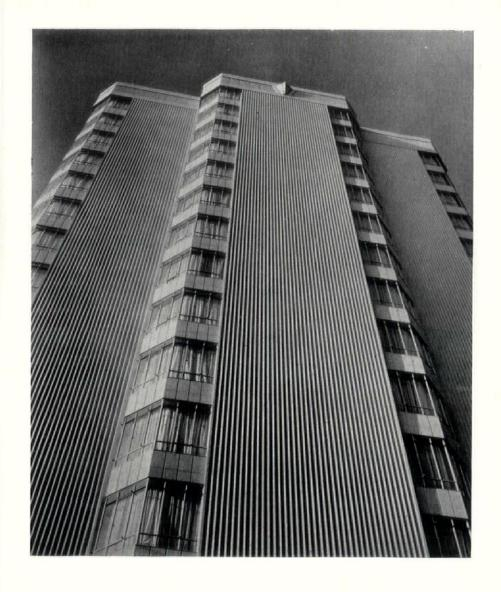
TEXTURE through form and scale obtained by using black corrugated iron as a form liner. Only two form sections were used, the lower one being removed when the concrete had hardened and replaced in perfect alignment above the upper one. Complete lack of joint lines visibly demonstrates the monolithic character of the construction. Edmond Meany Hotel, Seattle, Washington. R.C. Reamer, architect
