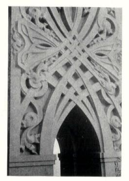
PRECAST in plaster moulds, this intricate detail from Baha'i Temple, Wilmette, III., is strengthened by a network of spot-welded reinforcing rods. The surface has been brushed to expose the aggregate. Louis Bourgeois, architect ONLY THE WINDOW and entrance trim of Grace Cathedral, San Francisco, is of precast concrete, the structure itself being monolithic. Strength, permanency and adaptability are significant characteristics
