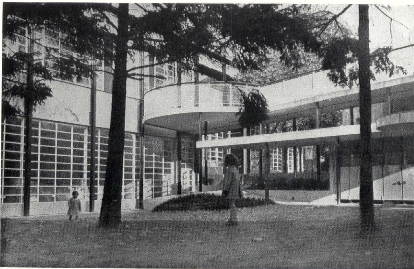
Looking toward the girls' two-story wing of the main building from the wooded central courtyard. The ramp which connects the dormitory floor with the roofs of the classrooms forms the roof of the connecting passages of the ground floor. A maximum of light and air is provided by the straightforward functional architecture which gains dignity through its very simplicity
