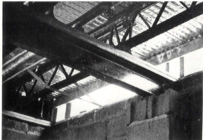
Structural units of the Reynolds System include plates, joists, floor slabs, and studs shown above and in several drawings, on page 92. Left: Detail of a typical assembly. Underside of floor slabs is a welded wire plaster base combined with metalized building paper
