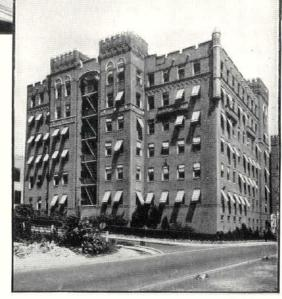
The Parkway Towers, beautiful East Yonkers apartment building. Eagle Insulation, installed early last spring for the year-round comfort of tenants, actually prevented costly damage a few months later when a roof blaze threatened to sweep the building. Fireproof Eagle mineral wool installed under the roof stopped the fire from spreading to the apartments below.
