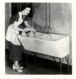
Crane Company, Chicago. It is of onepiece construction and is made of hard, durable porcelain. The corners are rounded for ease of cleaning and its glass-like surface is claimed to be unaffected by strong alkalies, dyes or acids (except hydro-fluoric). The double swinging spout faucet is installed above the rim of the tub to prevent back-siphonage. It may be had either in white or buff color and in both single and double compartments. **557M**
