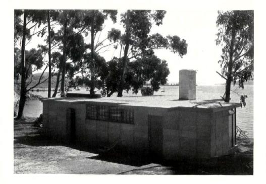
To withstand the strong winter winds of San Francisco Bay, the walls were constructed of Pacific Coast Aggregate Units (precast concrete blocks, 12 x 36 inches) — with reinforcing placed at the vertical joints and the space filled and poured as a column. The chimneys were built of the same materials. The floor is constructed of hollow building tile laid over a concrete slab. Crushed fire brick (the color of dried grass) and tar were used for the roof
