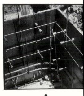
surface of which was square with the face of the wall and level in the direction of the wal Before the concrete hardened, this strip wa removed, permitting the next lift to be placed without feather edges and unsight irregular joints. Before placing a lift the concrete was well cleaned and covered with thick cement grout to insure a perfect bon
