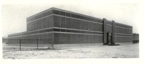
Built entirely of glass blocks in a new style of architectural design, this new research laboratory of the Owens-Illinois Glass Company at Toledo, Ohio, points the way to a new trend in industrial building construction. Above, is the entrance. The design over the door is aluminum depicting the old-time method of bottle blowing. At the top left, the building illuminated at night. Walker and Weeks, Architects.
