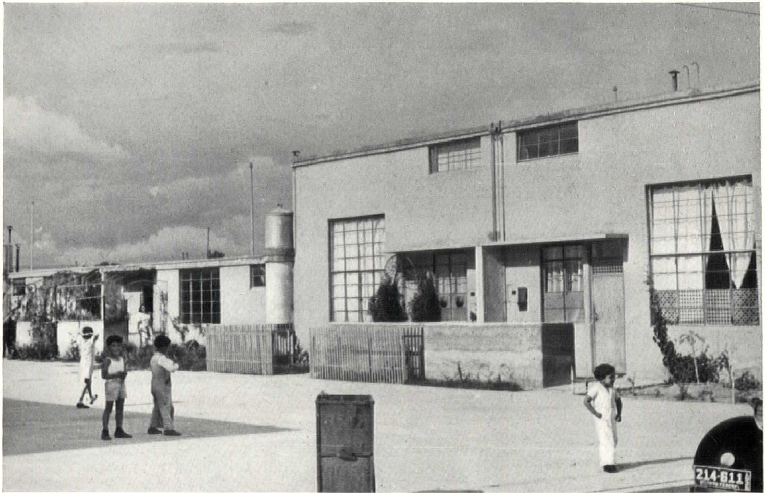
Adequate fenestration, while typical of all the government projects, is particularly noteworthy in the popular two-storied three-bedroom houses for large families (above). Immediately adjacent to Colonia Balbuena is a medium-sized private home, a maternity health station and a nursery school (center). Private enterprise has had less aesthetic success than the government in similar developments (below).
