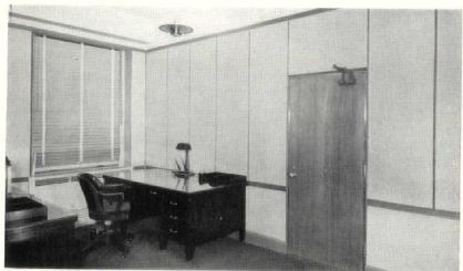
Private Office. Grey lacquered asbestos board panels carried around windows and exterior walls producing a uniformly attractive effect on all four walls of the room. Lacewood base, chair rail, cap mould, door and division strips.
