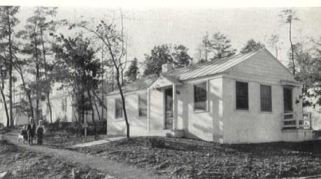
Four-room houses of cinder block (Type A) with paint finish. Floors are concrete slabs and roofs of metal. They are vermin and termite proof and also fire-resisting. Thirty such houses, with numerous exterior variations, were built
