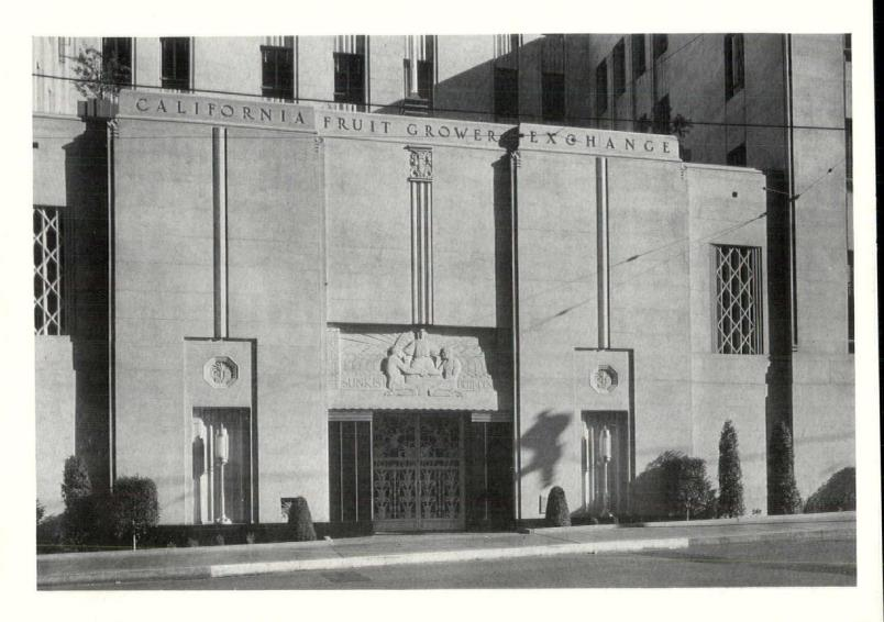
The garage surrounds the main foyer on the ground floor. The large board room without windows on the second story results in a unity of mass at the main entrance. Concrete forms were constructed of plywood in panel sizes. They were rigidly braced to assure exactness of surface in both directions. After stripping the surfaces were stoned and washed down to a uniform color and texture. Spandrels were acid stained
