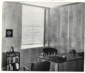
Private Office with natural colored lacewood wainscot, base, cornice and strips dividing wall into vertical panels applied on asbestos board partitions.
