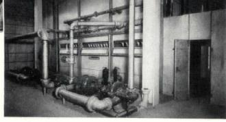
One of largest Dehumidifying Air Washers ever installed...a Sturtevant. 32 feet wide...16 feet high...21 feet, 9 inches long. Located at Ohio Match Company, Wadsworth, Ohio.
