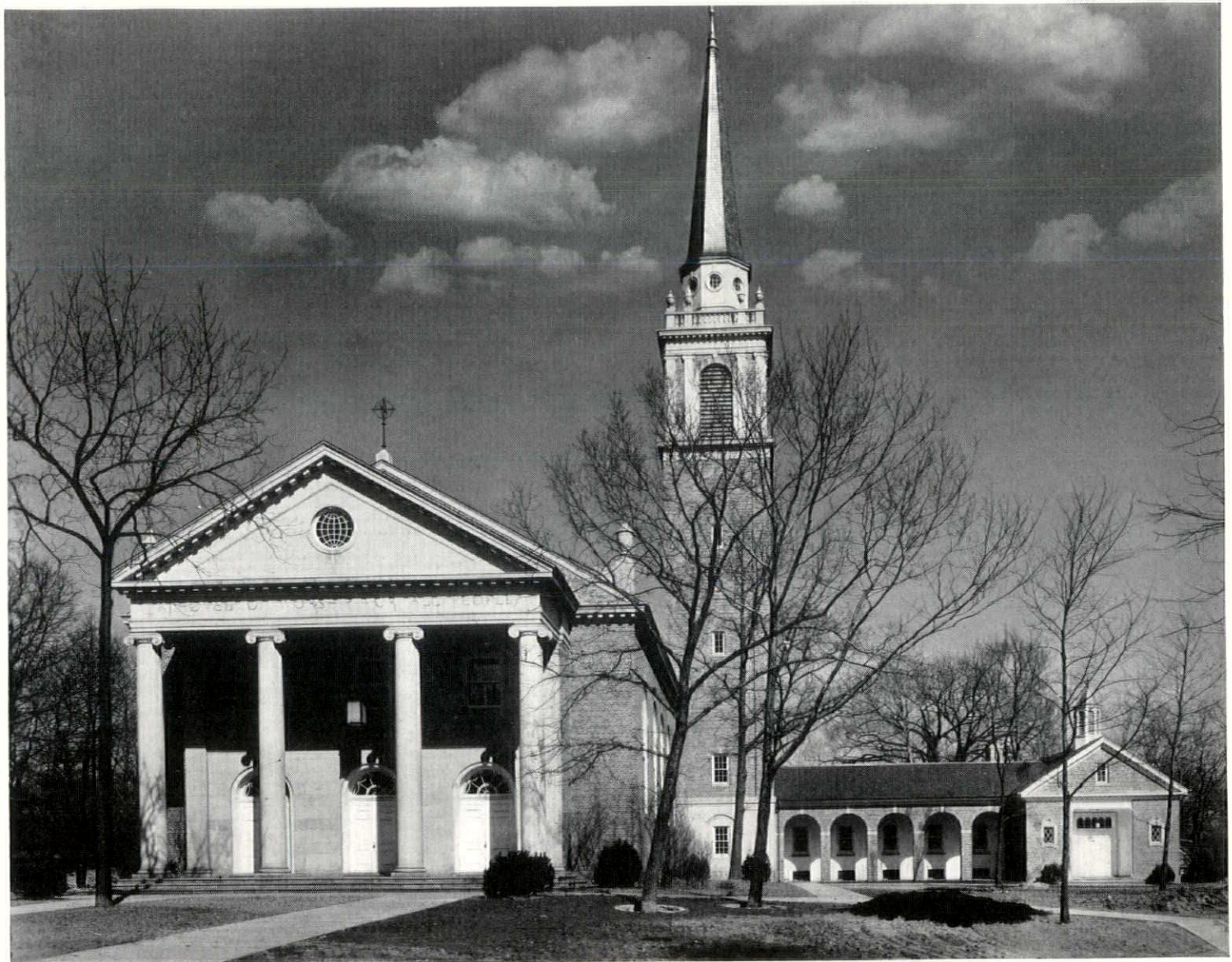
WINNETKA CONGREGATIONAL CHURCH, WINNETKA, ILLINOIS AYMAR EMBURY 2nd AND JOHN LEONARD HAMILTON, ASSOCIATED ARCHITECTS
