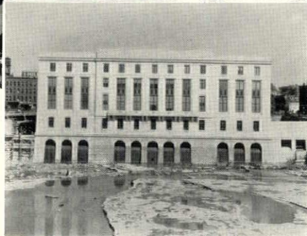
Rear view of Rundel Memorial Library, the first unit in Rochester's new civic center which will be built beside and over the Genesee River. More than 100,000 bd. ft. of Armstrong's Corkboard was used.
