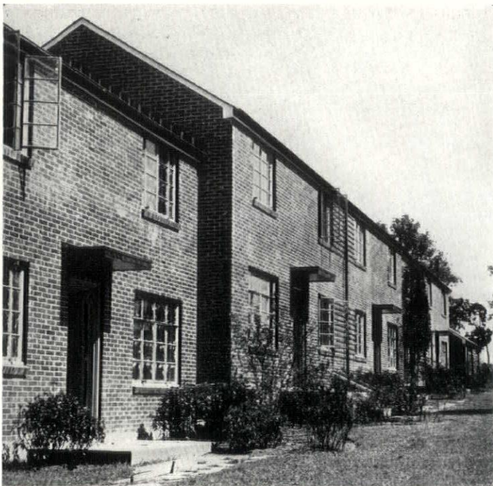
At left, a typical group in brick veneer construction, a detail section of which is shown below the photograph
