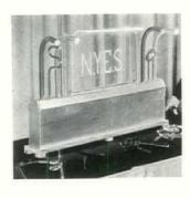
Lucite, a new crystal clear plastic by E. I. duPont de Nemours & Co., New York, transmits light around bends as was shown in a demonstration recently given by Mr. Harold Payne before the New York Electrical Society. Electric light bulbs were placed in a box on a table, below several rods and a sheet of Lucite The light was seen to travel
