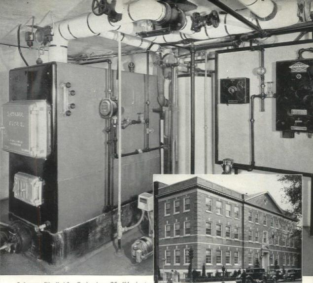
Boiler room of New York State Teachers Assoc., Office Bldg., showing left to right: Boiler with Oil Burner, Webster Boiler Protector, Control Valve, Variator, Webster Moderator Control Cabinet.
