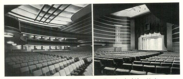
Kansas City Auditorium. Left: seats laid out in curved rows provide a maximum of comfort for spectators besides reducing wear on upholstery and strain on seats. Right: use of curved aisles introduces automatic staggering of seats without destroying alignment at aisles. Use of fully upholstered seats reduces acoustic problems
