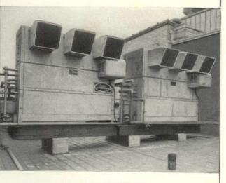
... CARRIER EVAPORATIVE CONDENSERS were located on the roof. Using less than 5% of the water required by water condensers or other type of water equipment, these efficient condensers solved the Leader Building's problem completely, without enlarging water mains.
