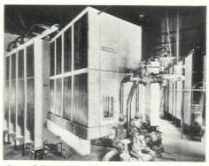
of the 14 Sturtevant Air Washers which have a total capacity of 980,500 c.f.m.
