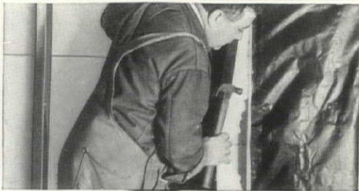
Showing stud application. Backed with heavy waterproof paper, RED TOP STRIP WOOL is easy to nail.
