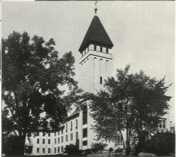
Main building of Villa Maria Academy, nationally famous school for girls, at Frontenac, Minnesota. Applicators: U. S. Roofing & Siding Co., St. Paul, Minnesota.
