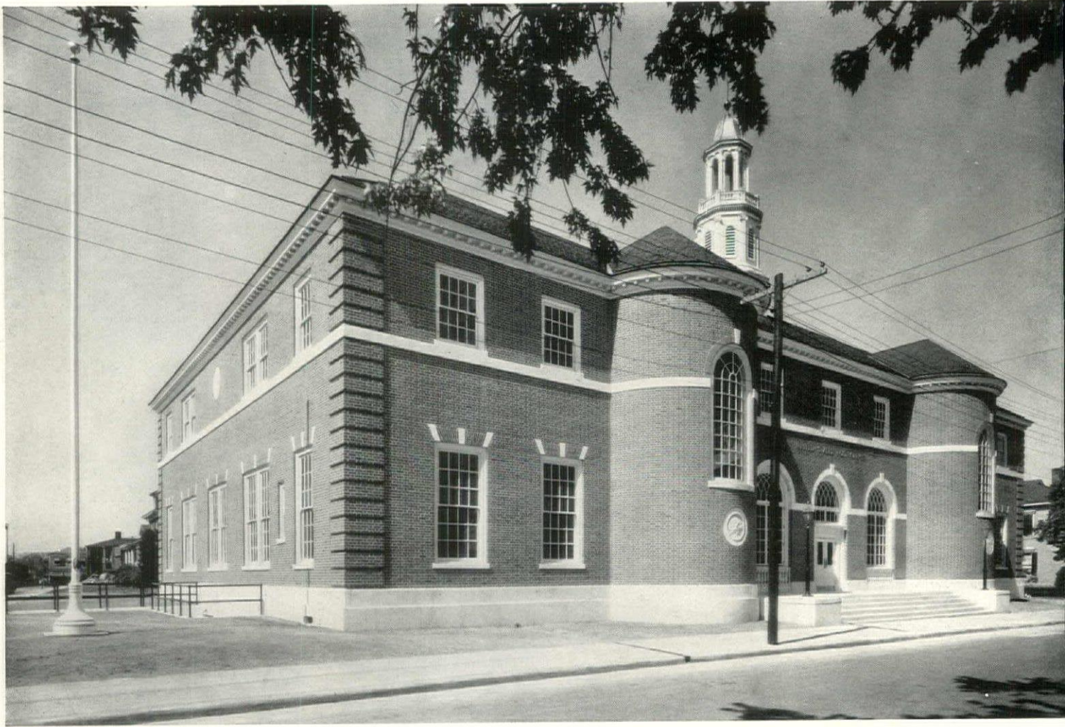
U. S. Post Office, Petersburg, Virginia Donald Anderson, Designing Architect, Procurement Division
