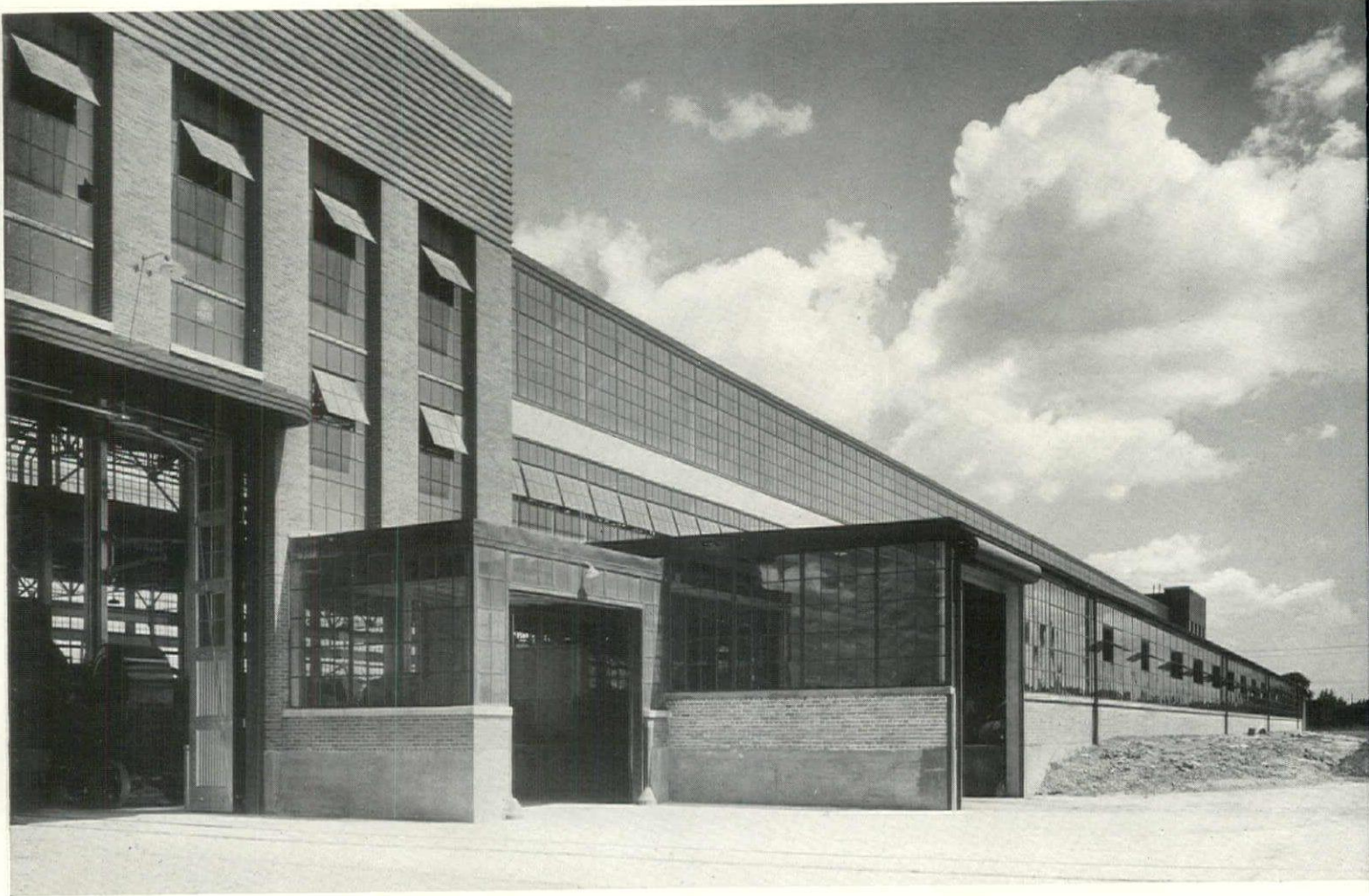
MACHINE SHOP, AMERICAN BLOWER CORPORATION ALBERT KAHN, INC., ARCHITECTS
