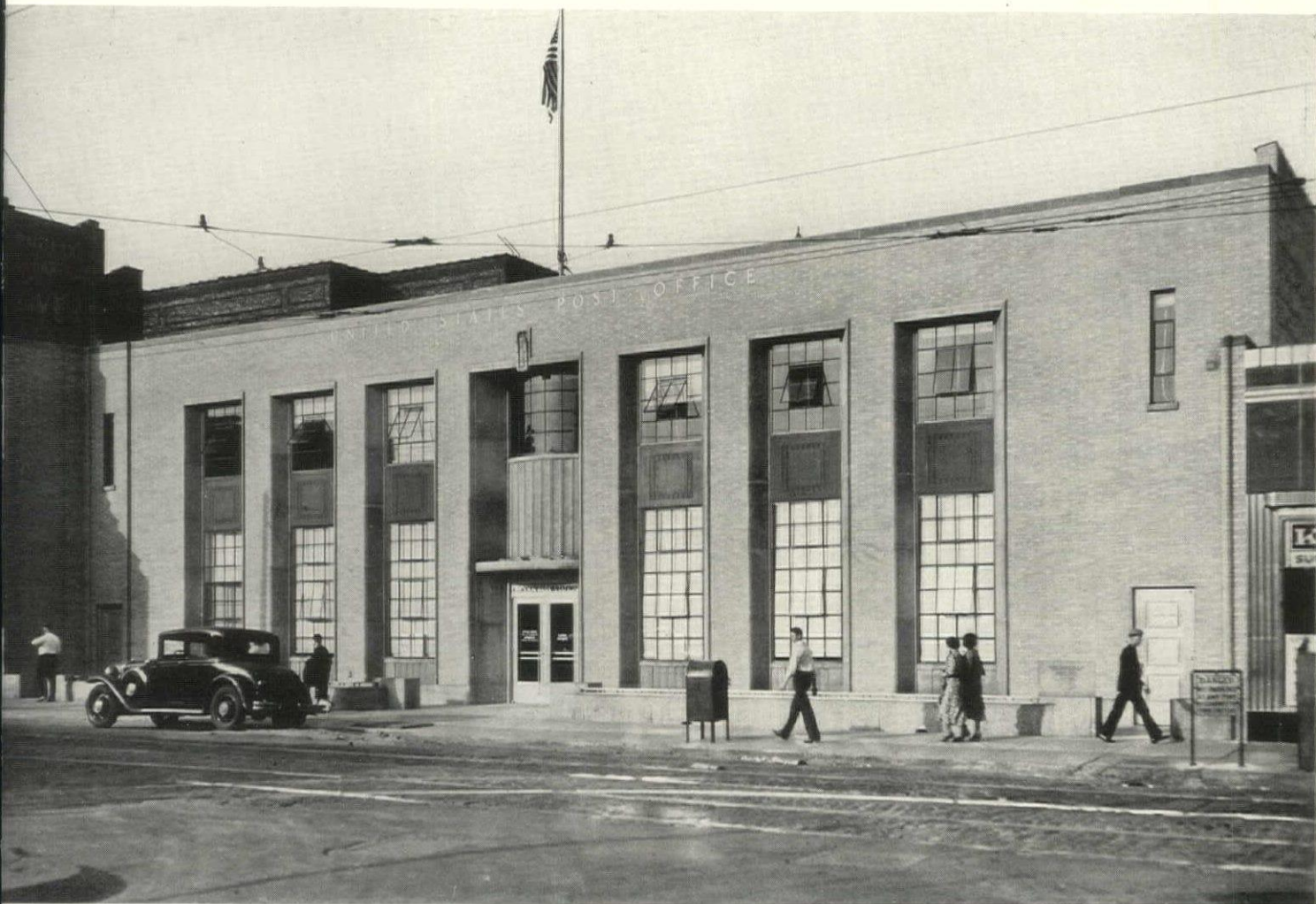
In Park Postal Station, Chicago, Illinois. Ward L. Cheney, Designing Architect, Procurement Division
