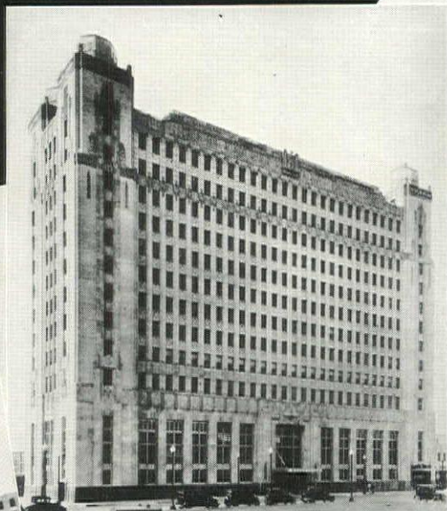
● Byers Wrought Iron specified in Texas and Pacific Passenger Station, Fort Worth, for all water pipe above ground, all steam piping below first floor and in tunnels, and all steam return piping below fourth floor.
