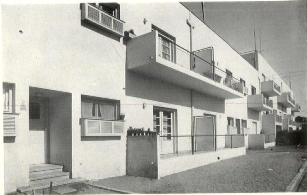
WORKERS' DWELLING HOUSES, RAMAT GAN J. NEUFELD AND I. DICKER, ARCHITECTS
