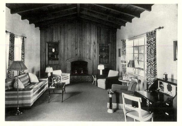
All interior trim, including ceiling and fireplace wall paneling, is of cypress. Flooring is of oak. The second floor exterior wall on the garden side (below) is of frame, sheathed roofing felt, metal lath and stucco. Porch flooring is of handmade Cuban tile on concrete slab.
