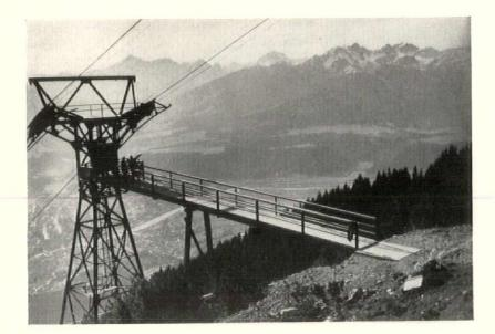
**REST STOP**... There are four intermediate stops between the first and second stations. They are of the simplest possible nature, consisting of a railinged wood platform.
