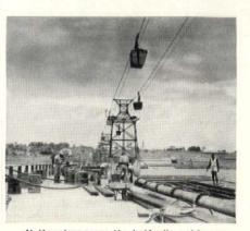
It then traverses the half-mile cableway that leads to the loading pier —
