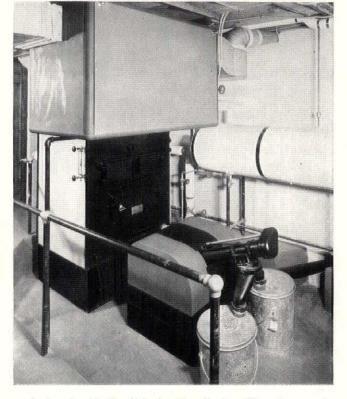
Anthracite Air Conditioning Installation. Note Automatic Anthracite Burner—feeds fuel automatically—removes ash to sealed containers.
