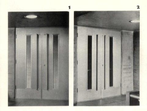
In rooms which house extremely sensitive instruments, this louver-paneled door is bucked up by interchangeable glass wool filters, composed of standard 6" wide units, for which the width of the louver panel was designed. The door is made in either aluminum or enameled steel.
