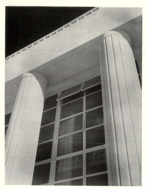
Exterior walls are of painted brick, limestone and cast stone. Partitions and insulation are of terra cotta. The interior finish is of plaster and terra cotta. Foundations are of concrete while concrete and tile are used for roofing. Floors are concrete, ceramic tile and terrazzo. Windows are steel.
